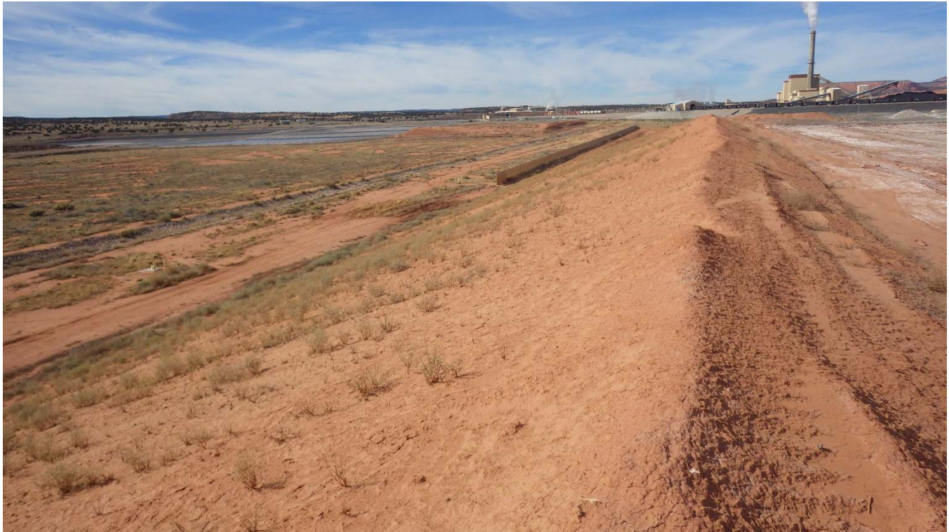
Photograph 2: Typical Embankment Crest Condition
