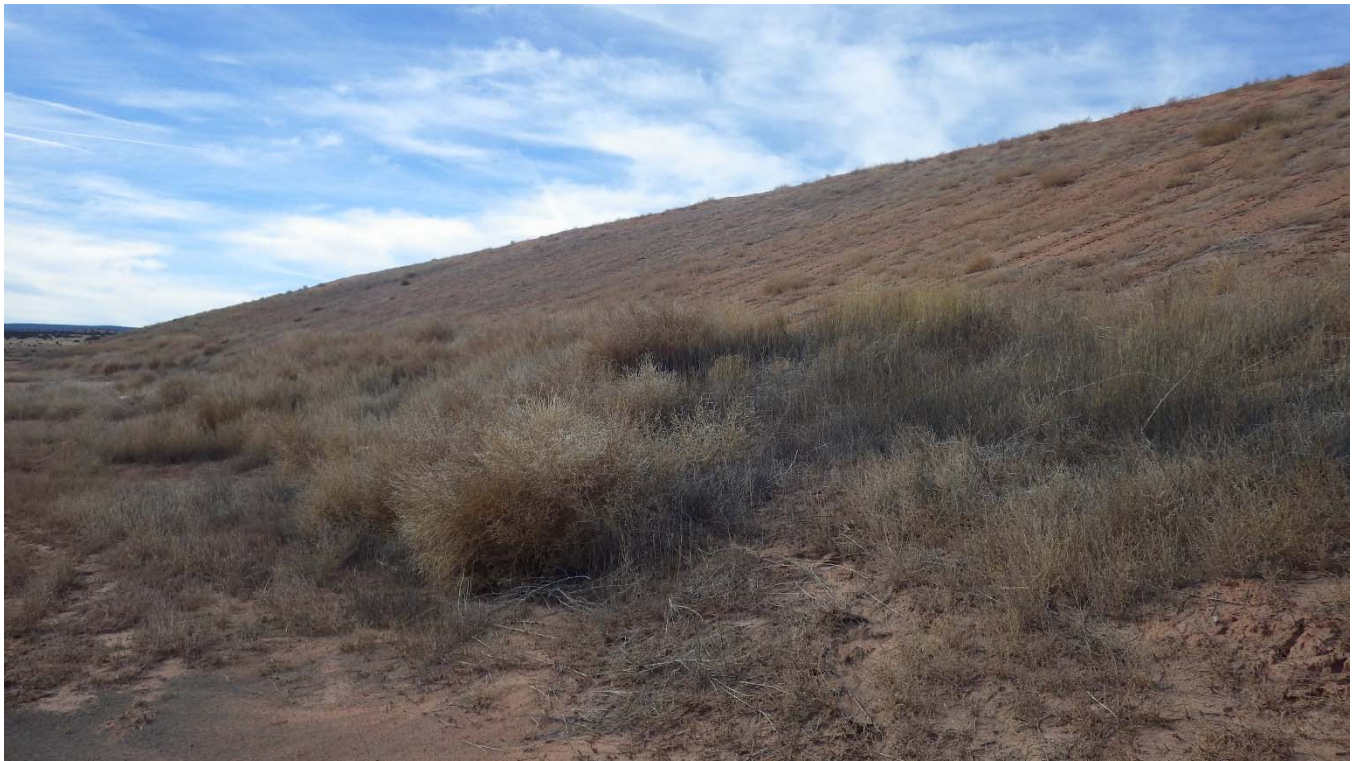
Photograph 4: Typical Embankment Toe Condition
