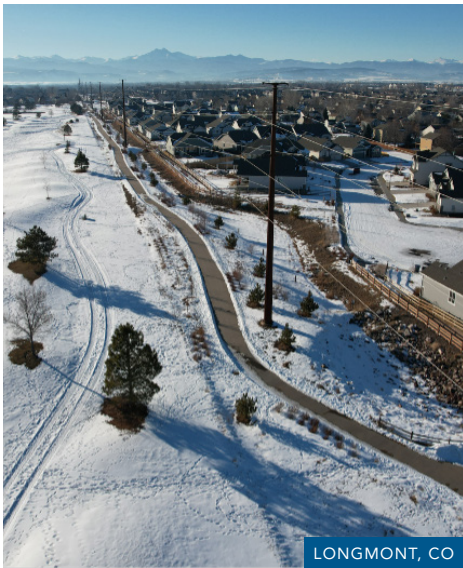
Facilities: Del Camino Tap-Meadow 115kV & Fordhan-Fort Saint Vrain 230kV Transmission Lines
