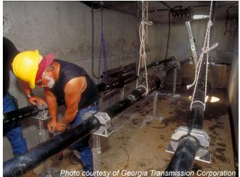
Working on underground lines in typical 8x8x24 foot manhole
