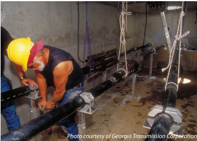
Working on underground lines in a typical 8' x 8' x 24' vault
