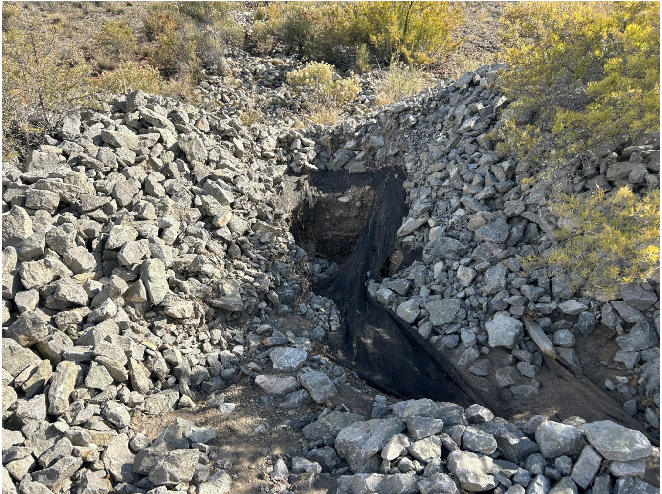
Photograph 8: Downchute Channel Erosion
