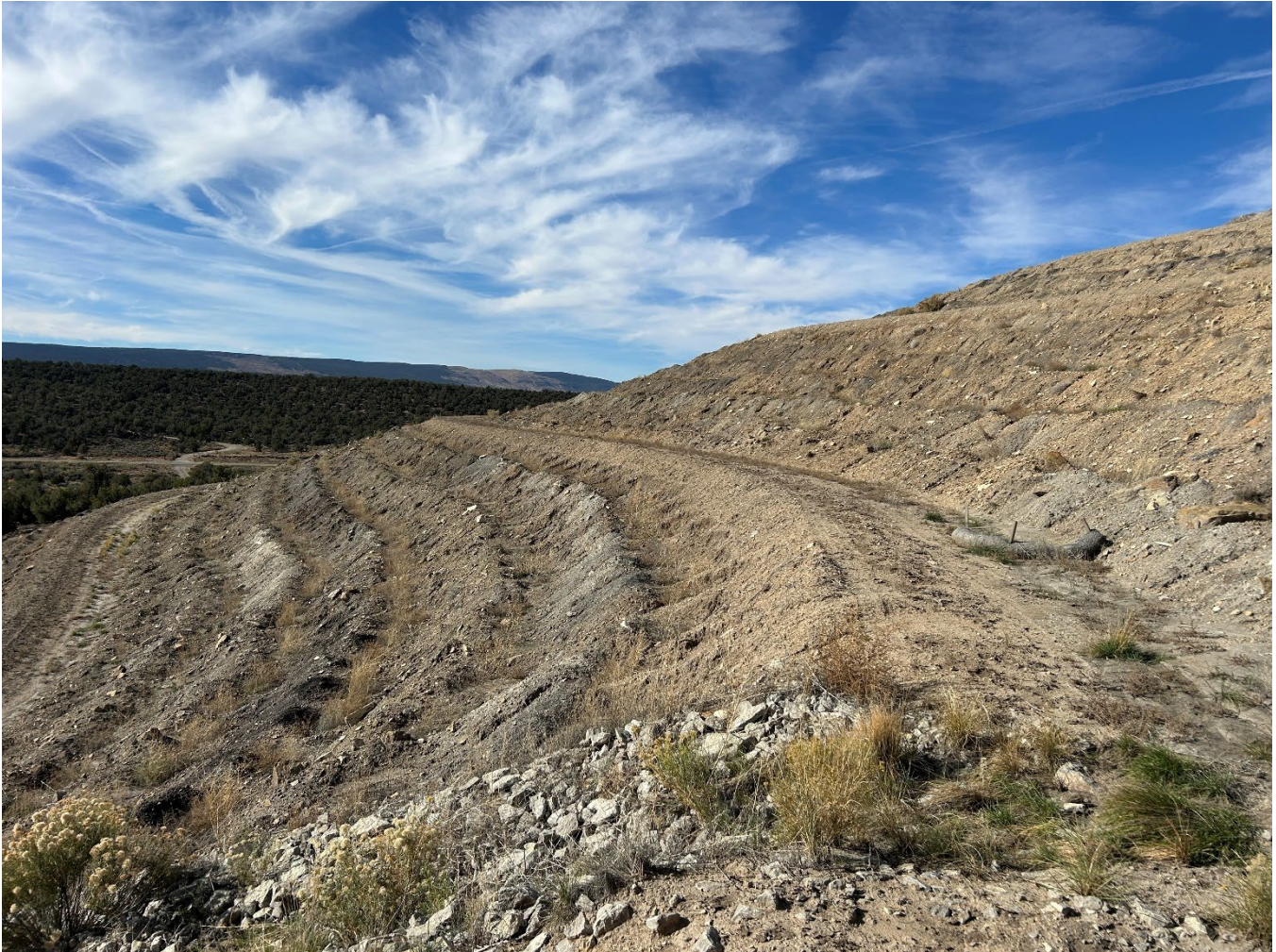
Photograph 4: Typical Condition of the South Embankment Slope
