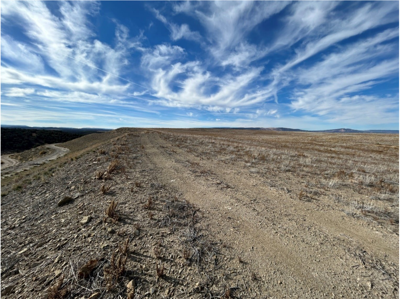
Photograph 2: Typical Condition of the Embankment Crest
