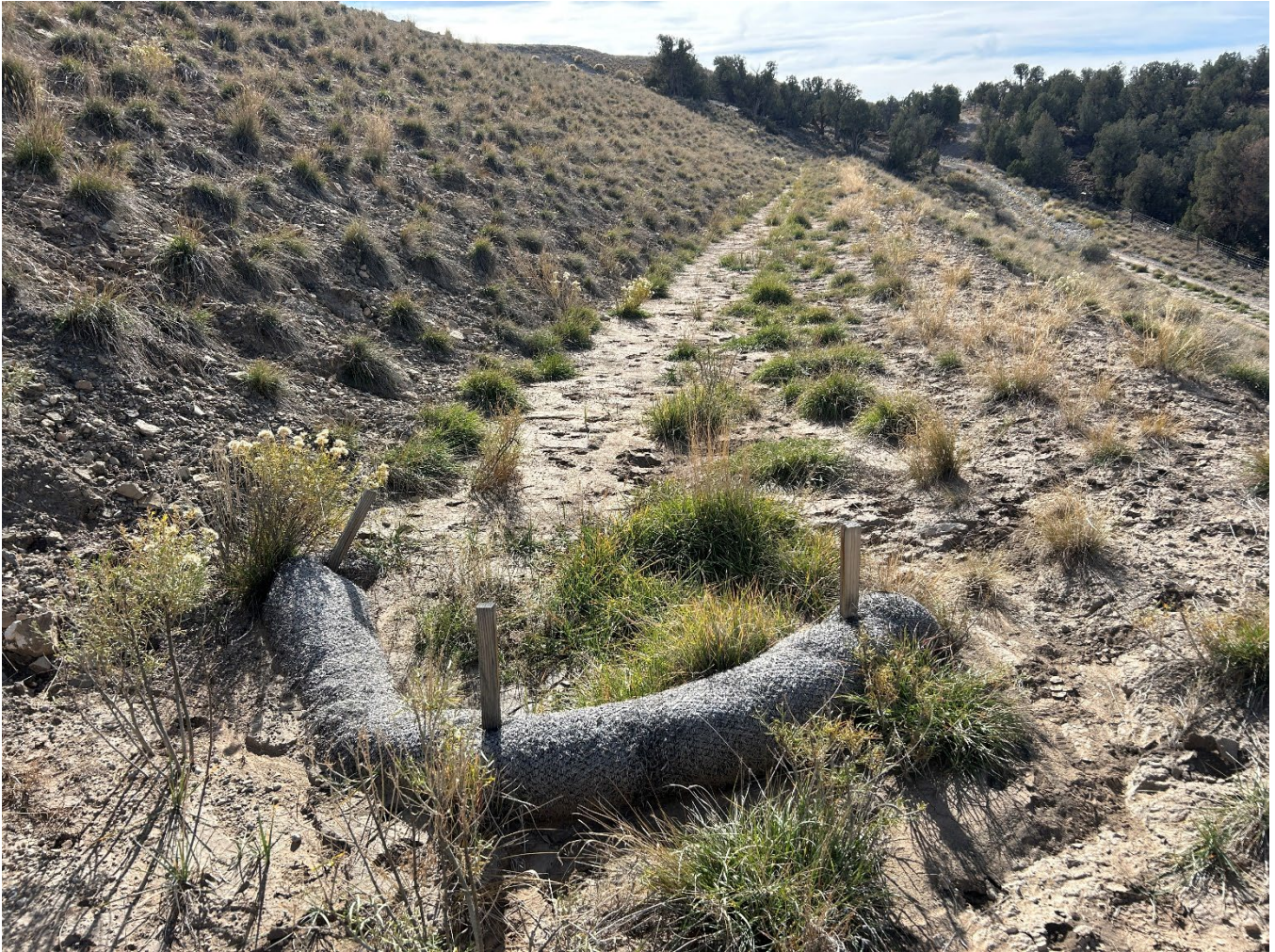
Photograph 9: Typical Condition of Terrace Channels
