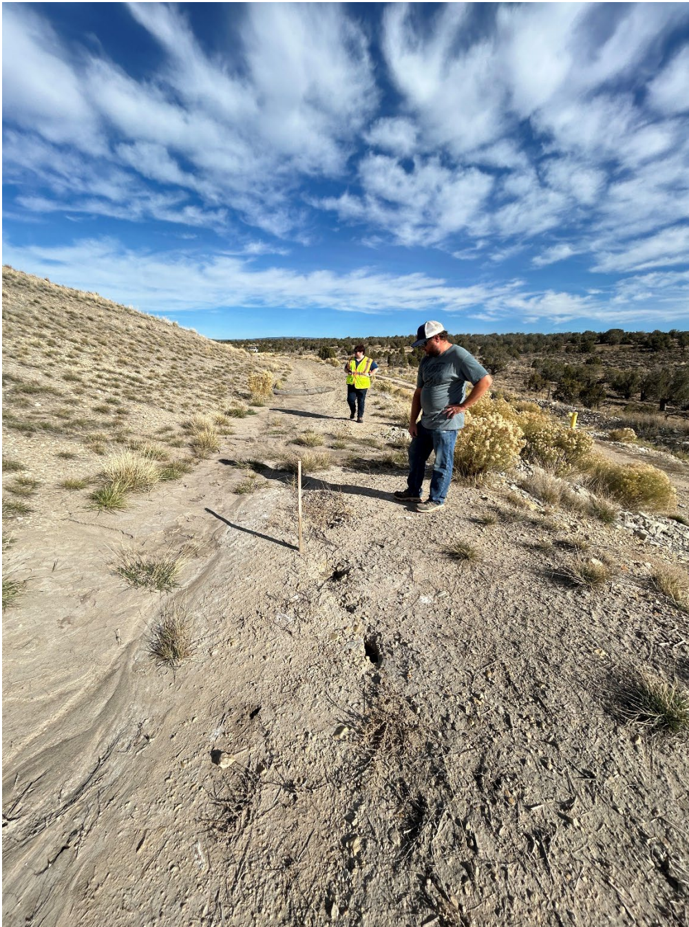
Photograph 3: Crack in an East-facing Side Slope Terrace Channel
