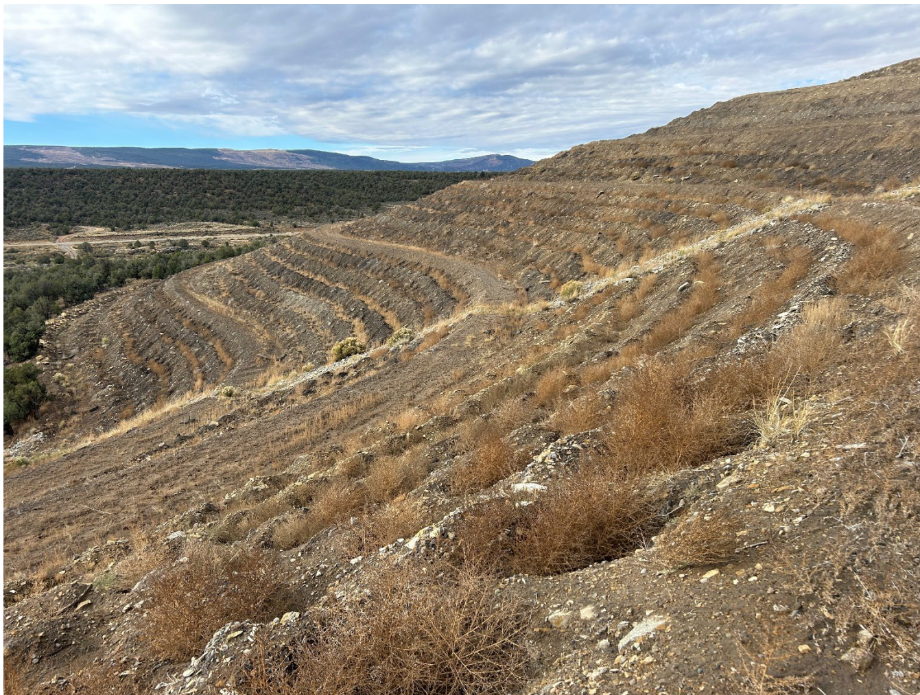
Photograph 3: Typical Condition of the South Embankment Slopes
