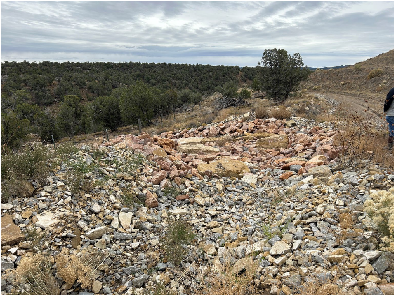
Photograph 9: Stormwater Outfall 07 (looking south)
