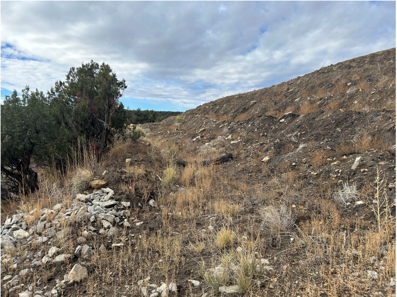
Photograph 5: Typical Condition of the Embankment Toe
