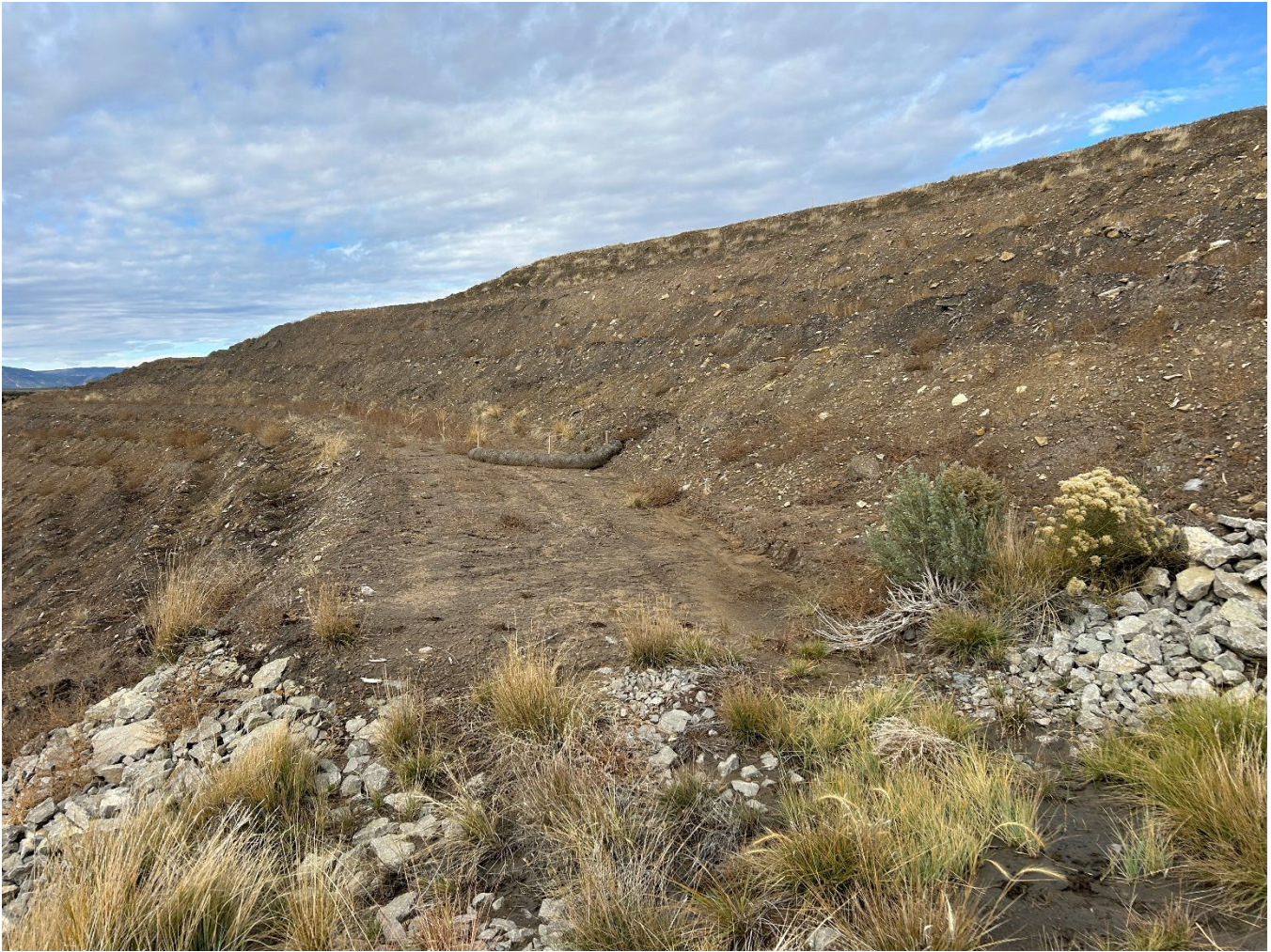
Photograph 7: Typical Condition of Terrace Channels
