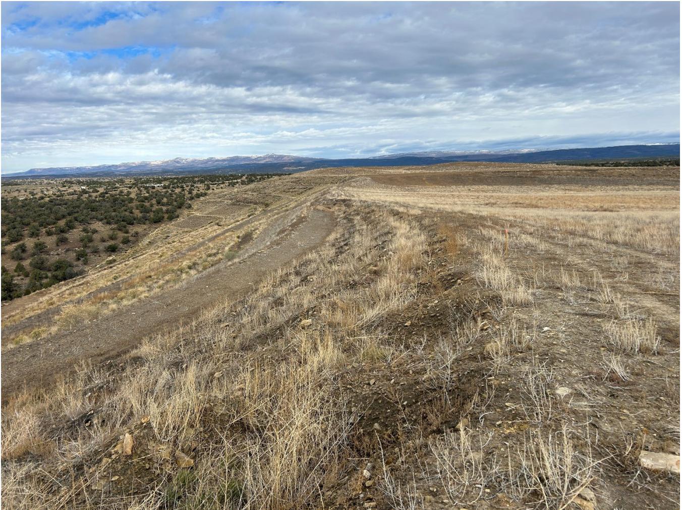
Photograph 2: Typical Condition of the Embankment Crest
