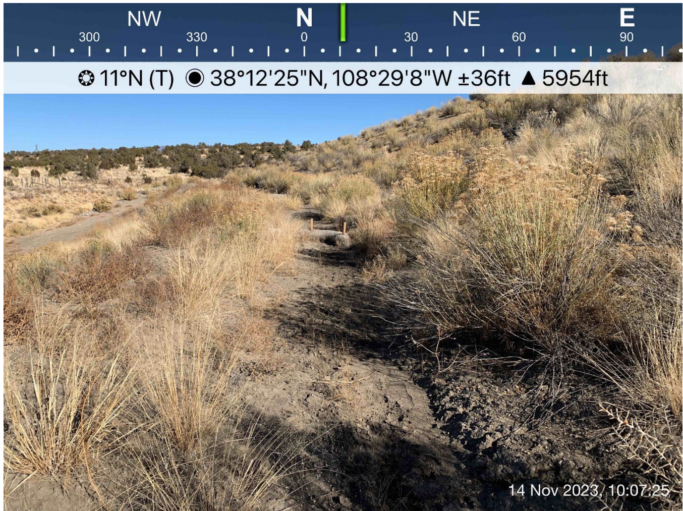
Photograph 5: Typical Condition of the Embankment Toe
