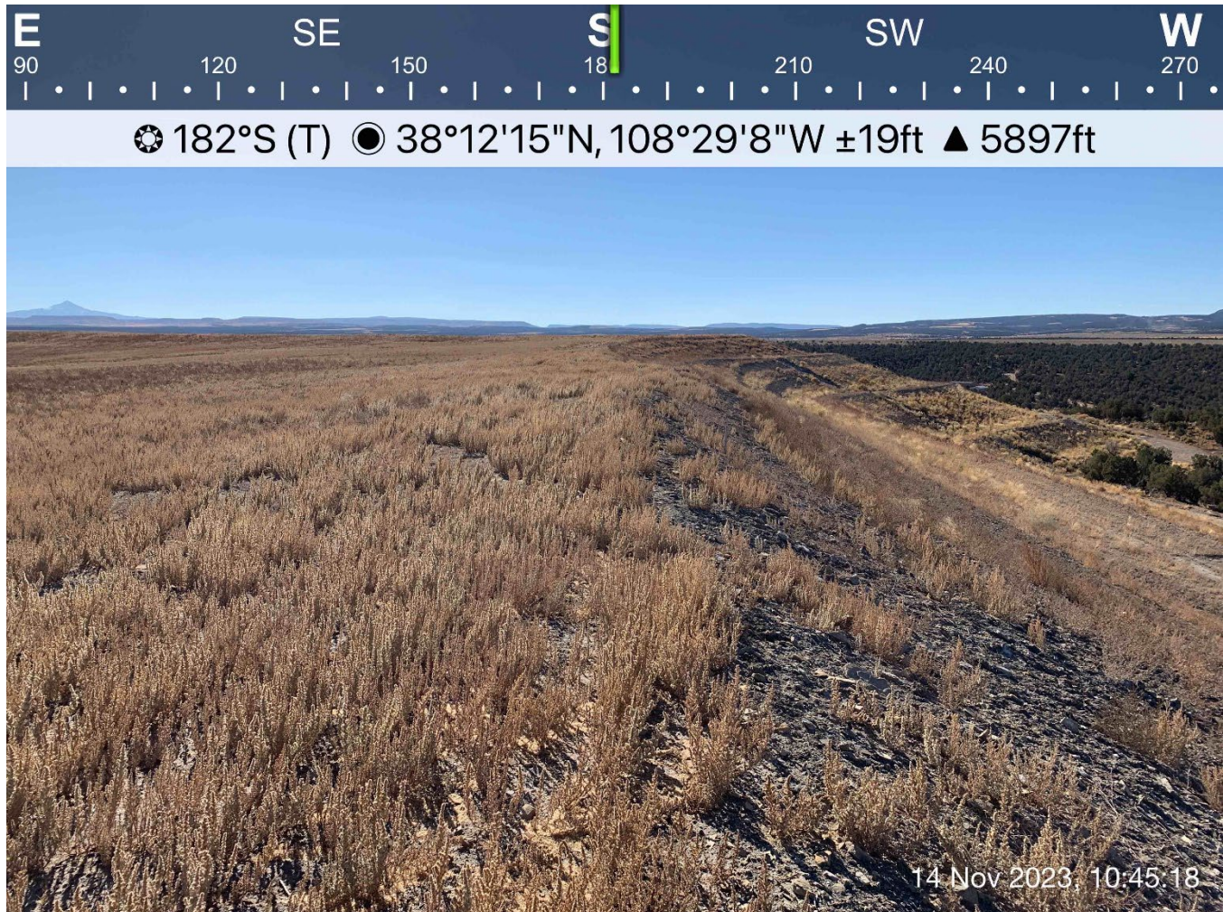
Photograph 2: Typical Condition of the Embankment Crest
