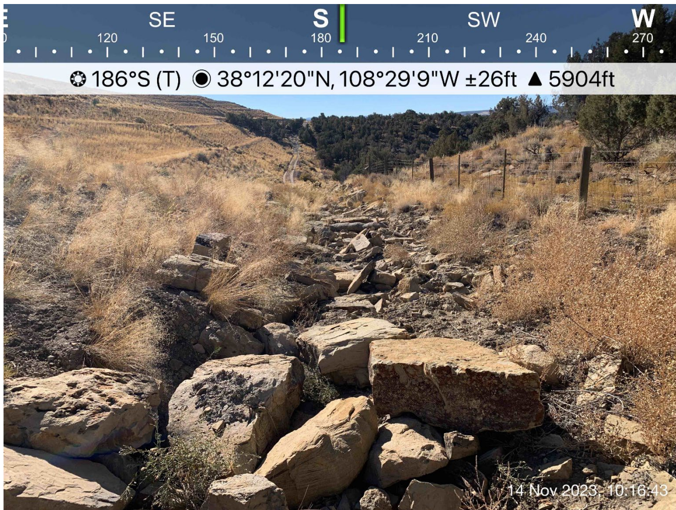
Photograph 8: Typical Condition of Perimeter Channels
