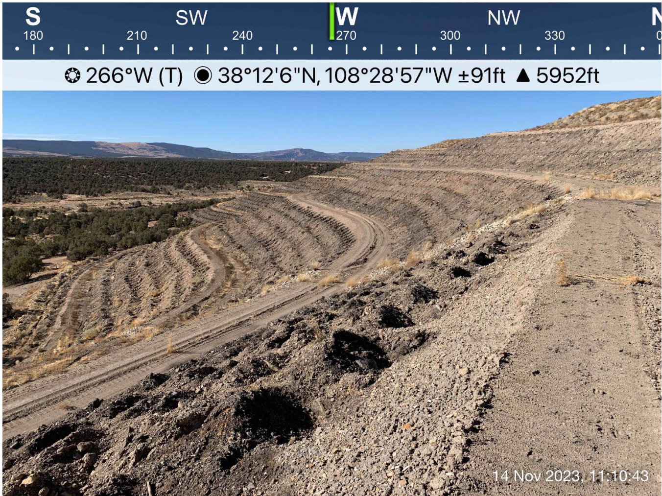
Photograph 3: Typical Condition of the South Embankment Slopes
