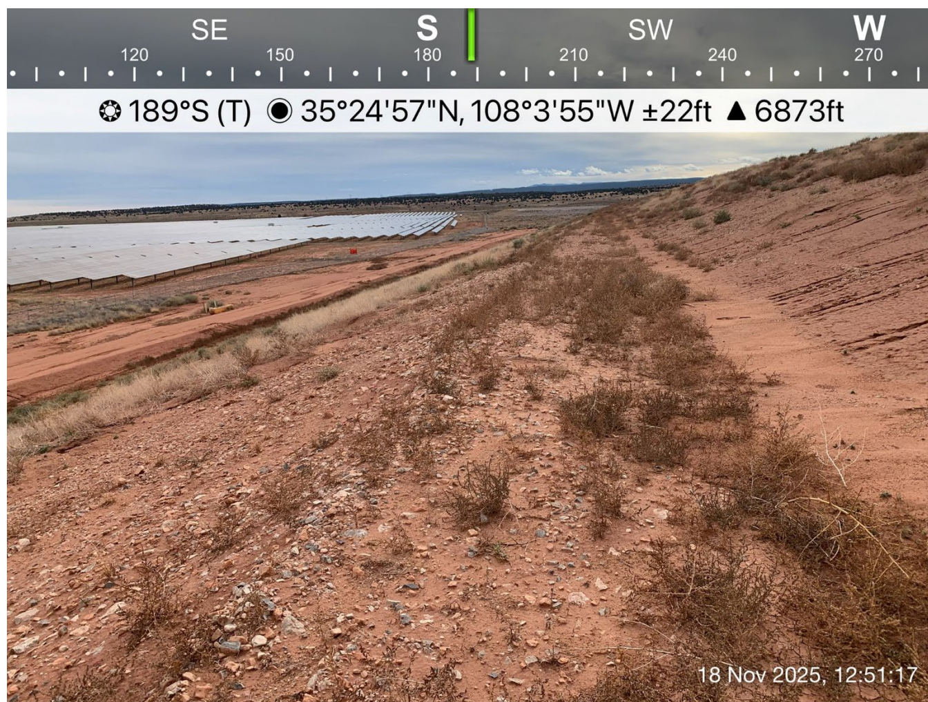
Photograph 9: Typical Condition of the Terrace Channels
