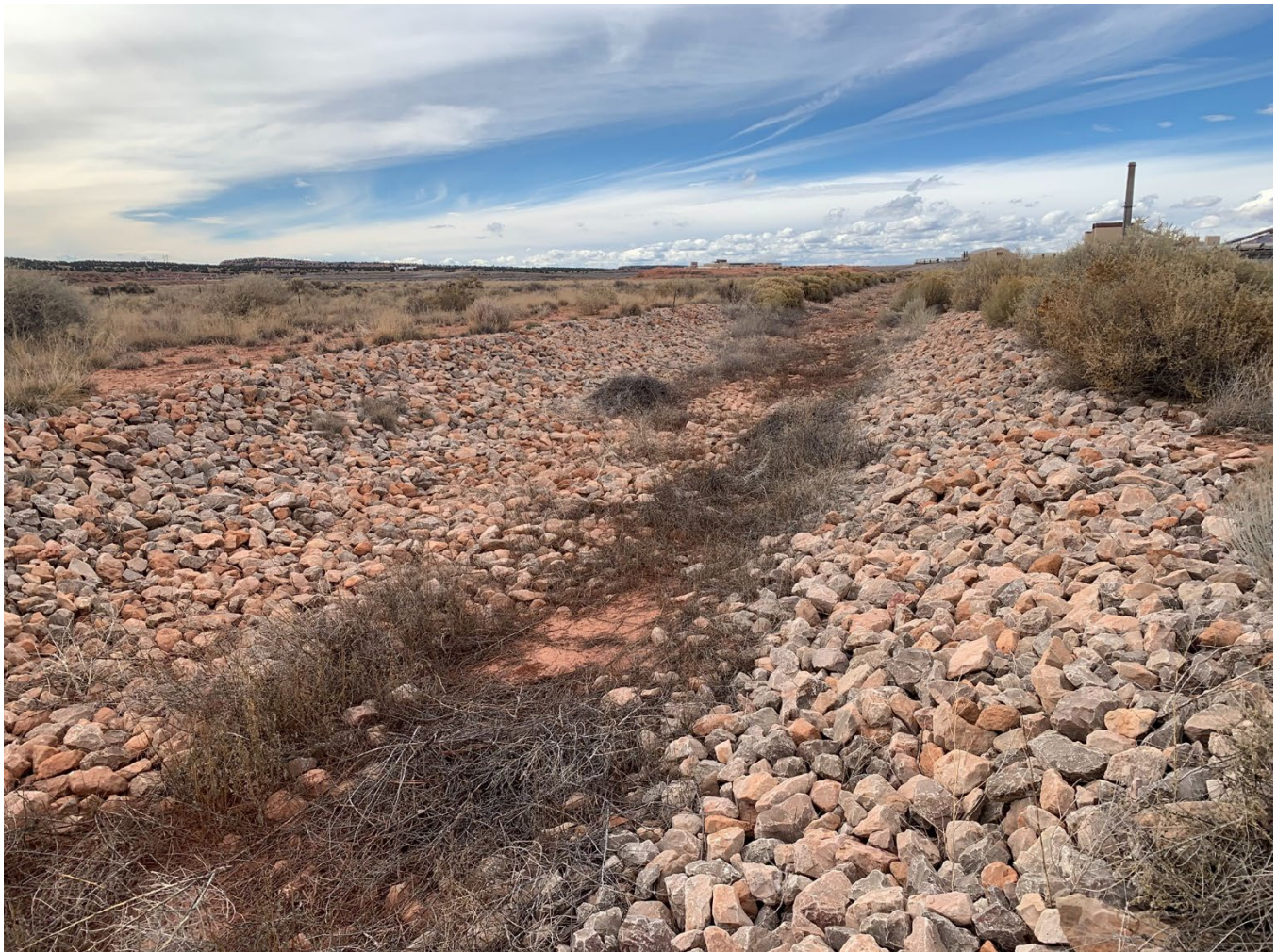
Photograph 8: Typical Condition of the Run-on Control Channel
