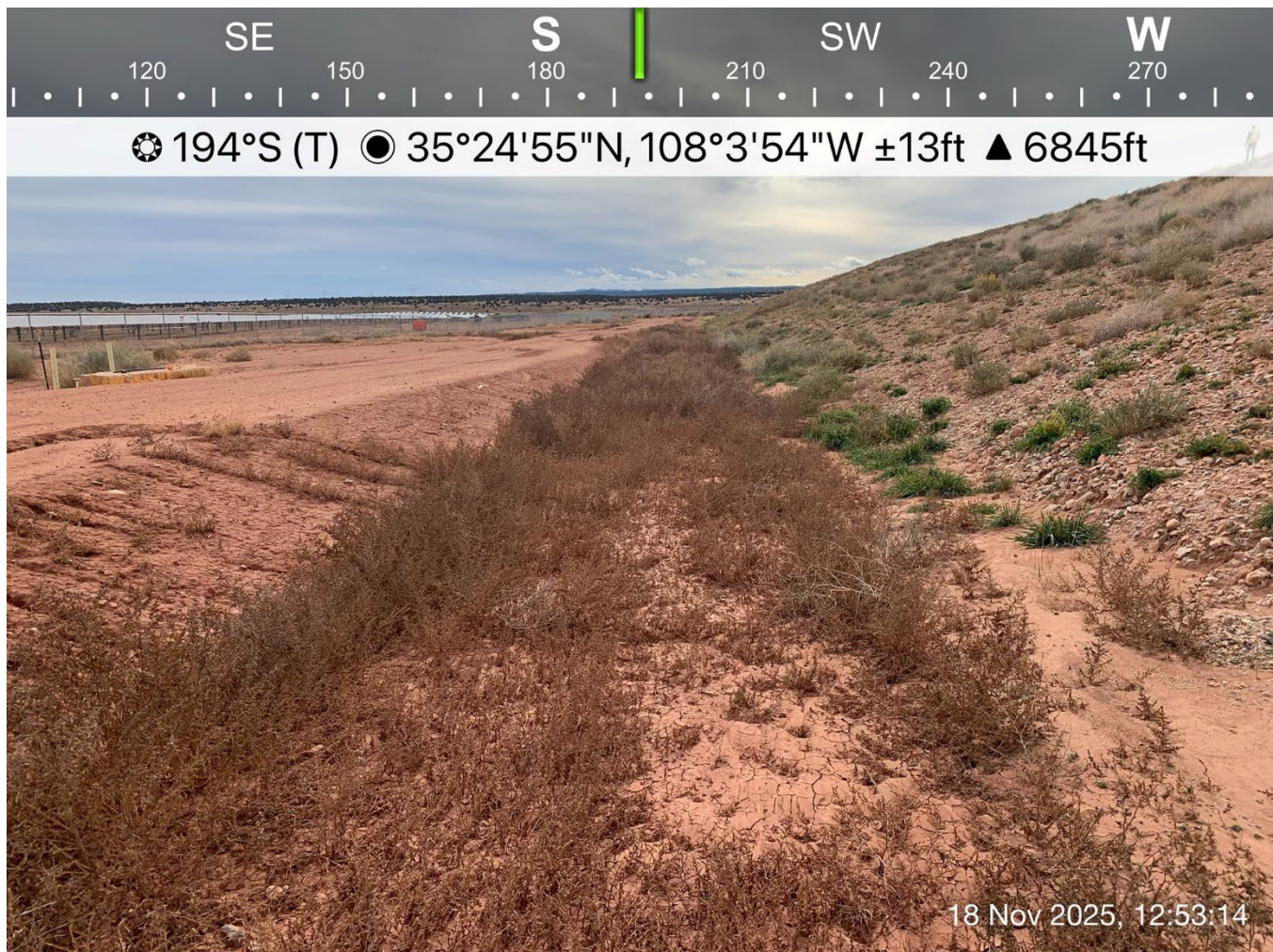
Photograph 7: Typical Condition of the Embankment Toe
