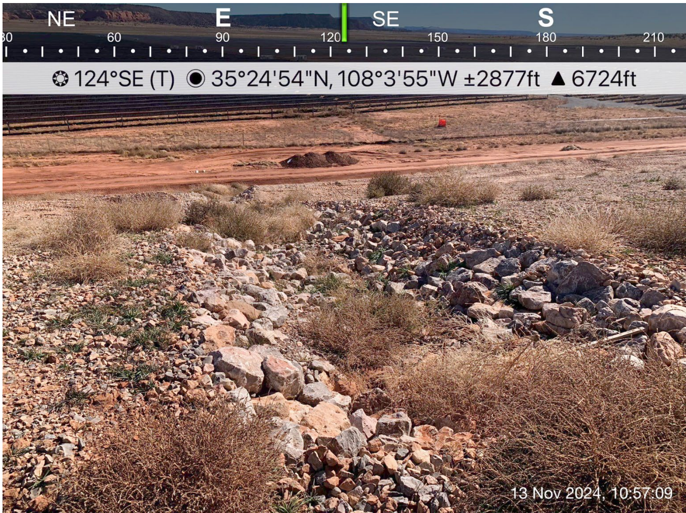
Photograph 11: Typical Condition of the Downchute Channel
