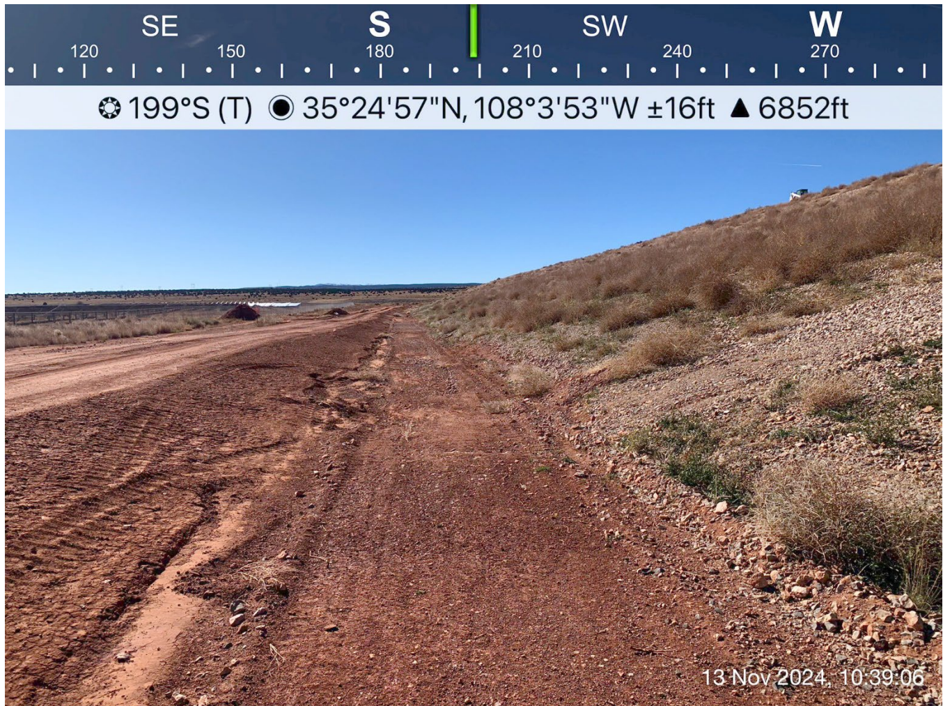
Photograph 7: Typical Condition of the Embankment Toe
