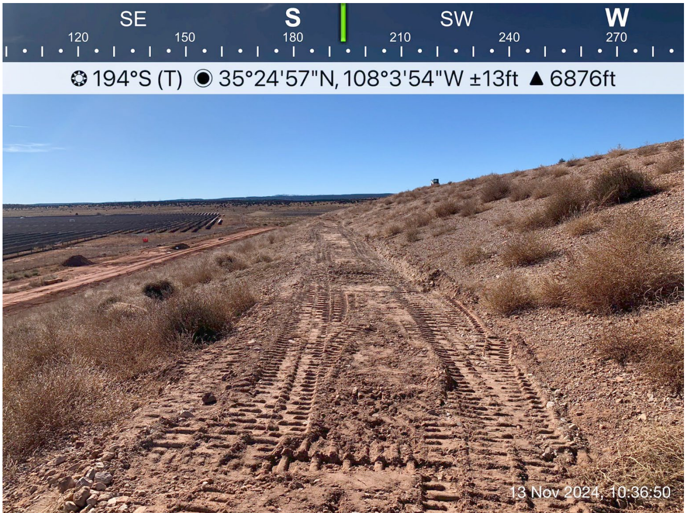
Photograph 9: Typical Condition of the Terrace Channels
