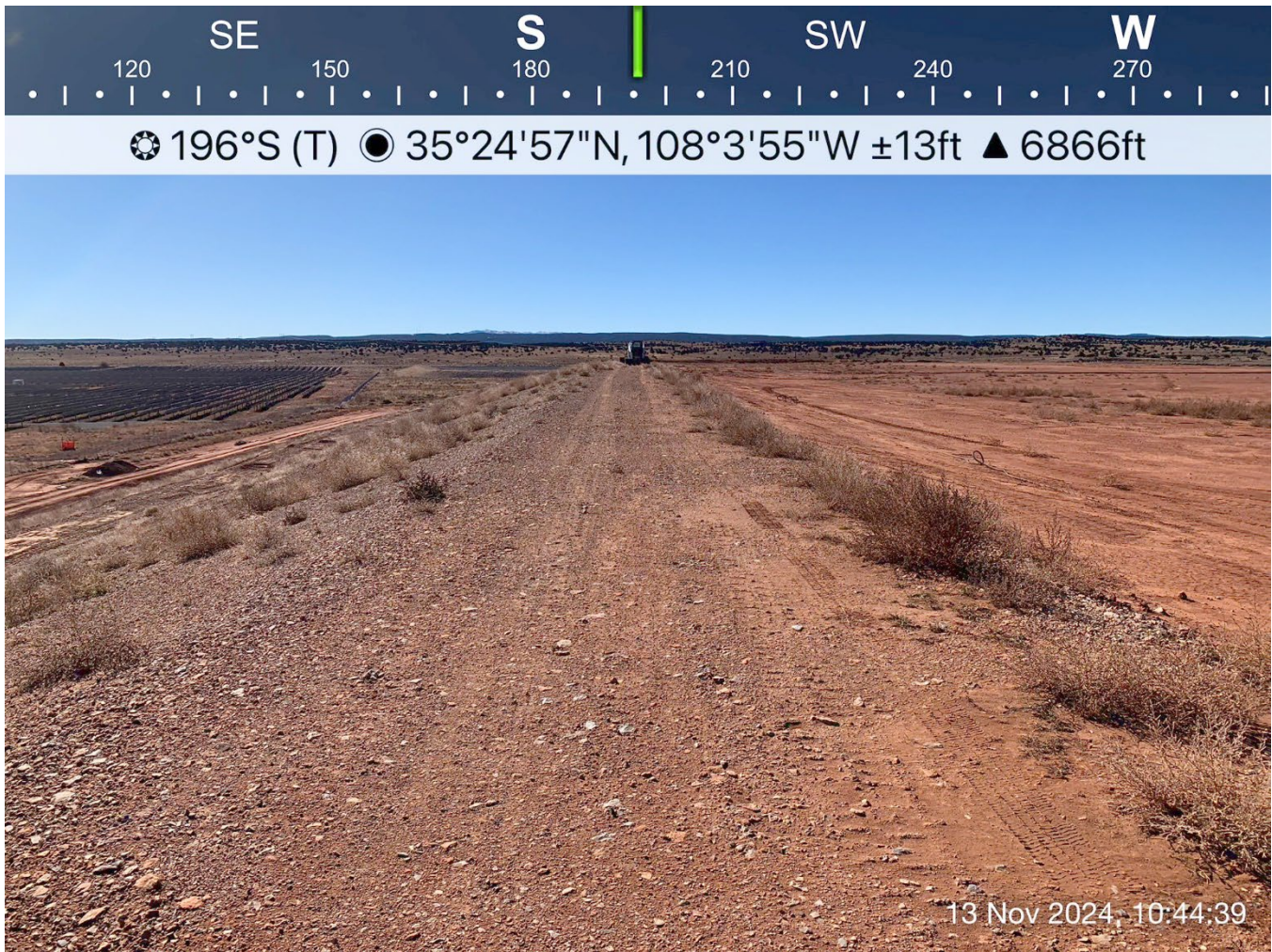
Photograph 4: Typical Condition of the Embankment Crest
