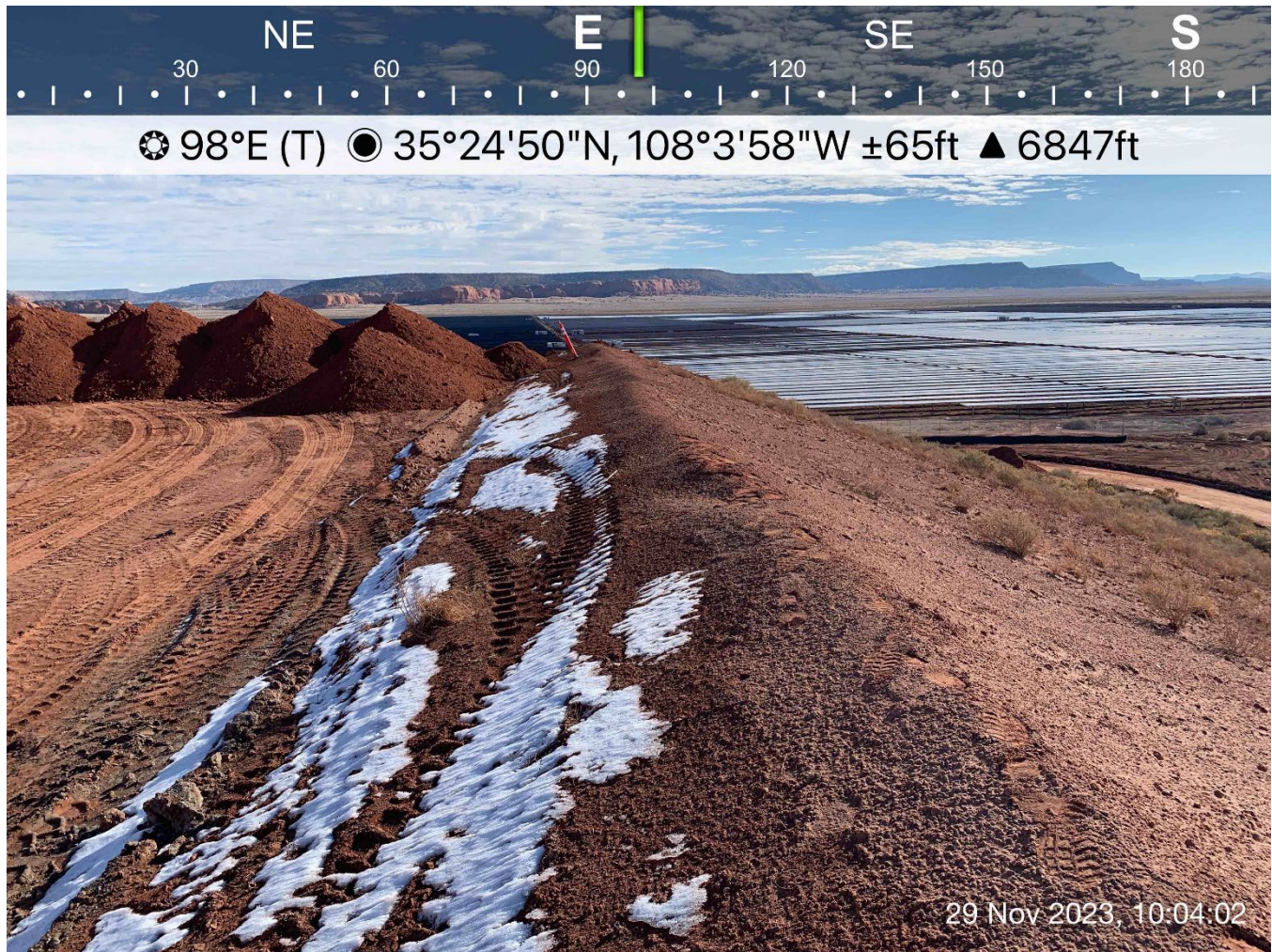
Photograph 2: Typical Condition of the Embankment Crest
