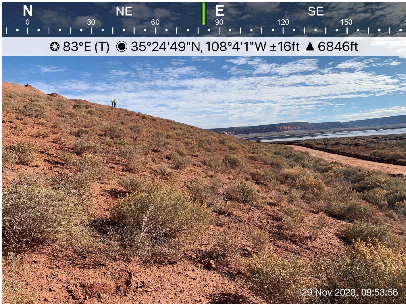
Photograph 3: Typical Condition of the South Embankment Slope
