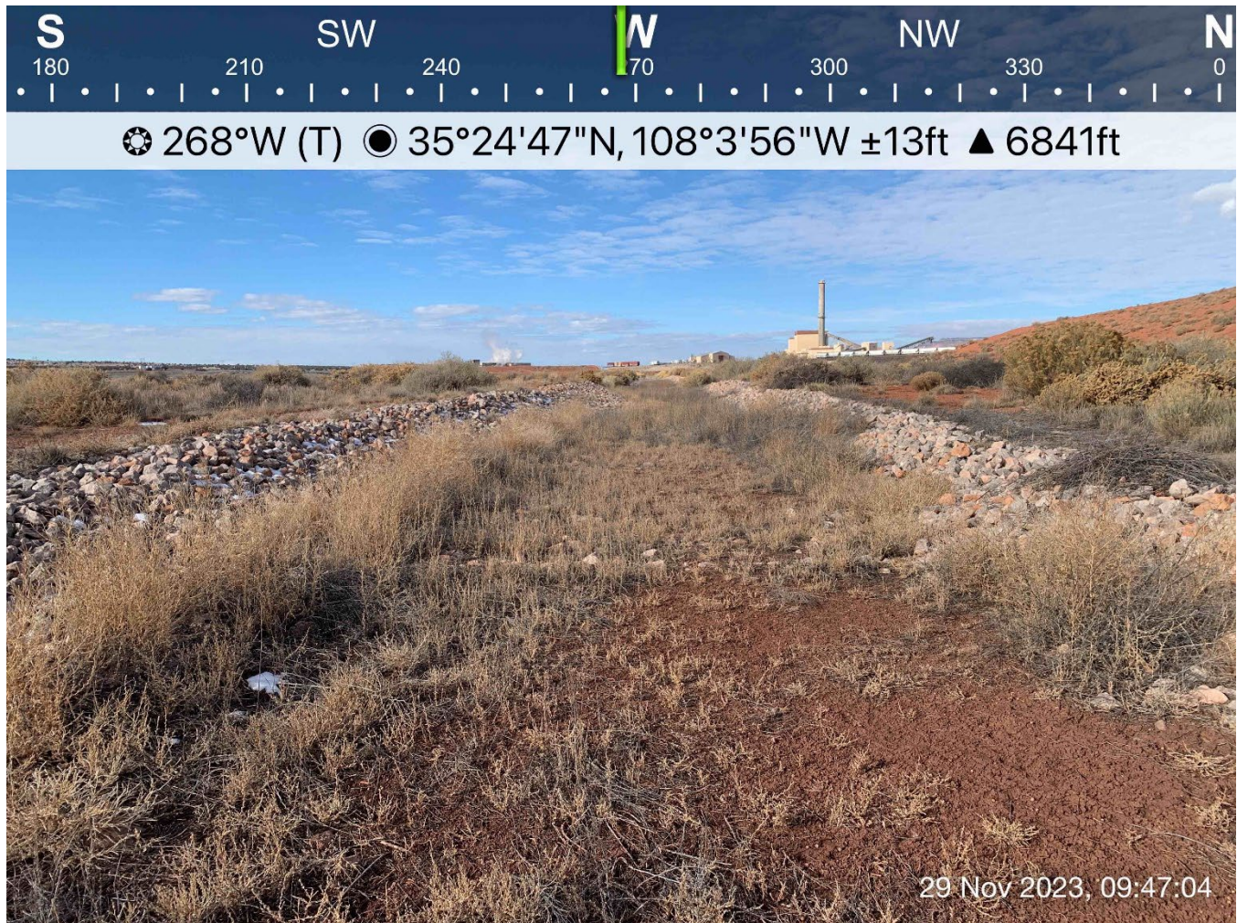
Photograph 6: Typical Condition of the Run-on Control Channel
