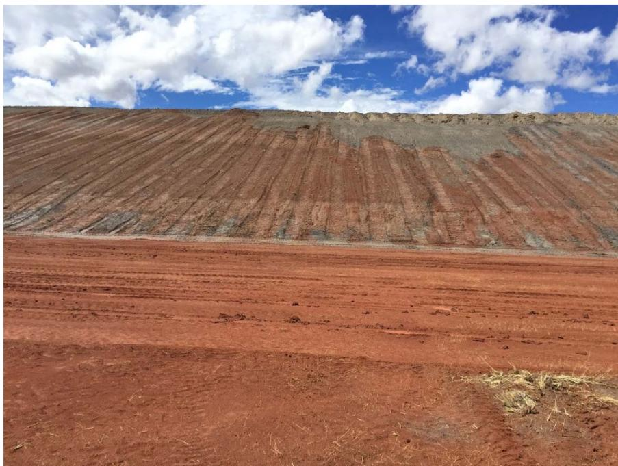
**Figure 4: Typical Embankment Toe Condition**
