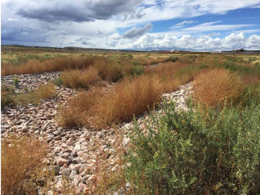
**Figure 5: Typical Storm Water Channel Condition**
