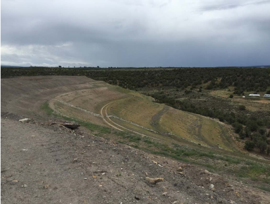
Figure 3: Typical Embankment Slope Condition
