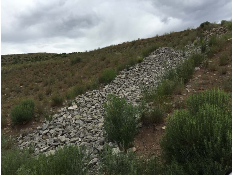
Figure 6: Typical Downchute Channel Condition
