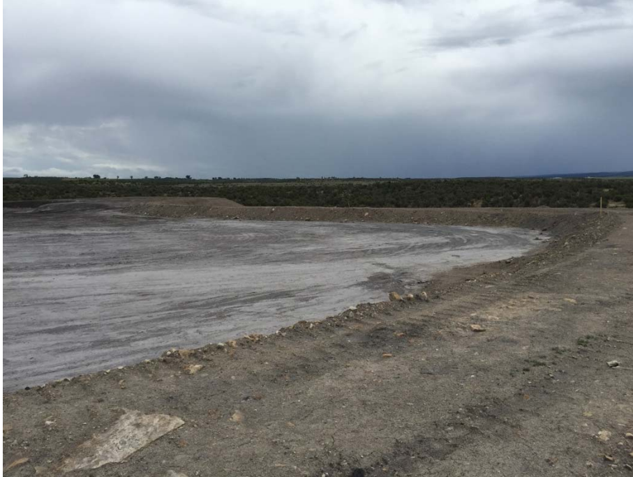
Figure 1: Typical Ash Deposition Area Condition
