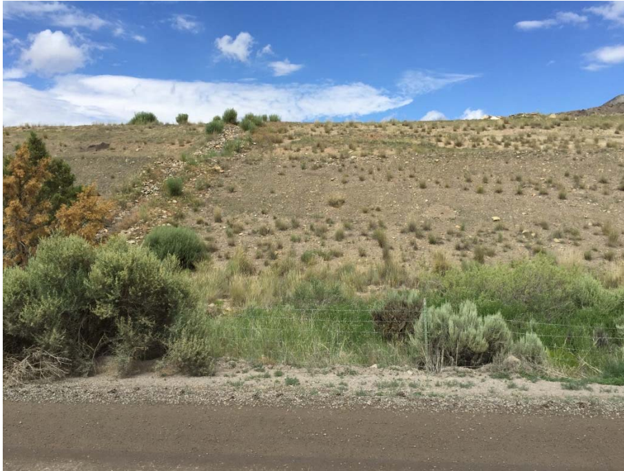
Figure 5: Typical Embankment Toe Condition
