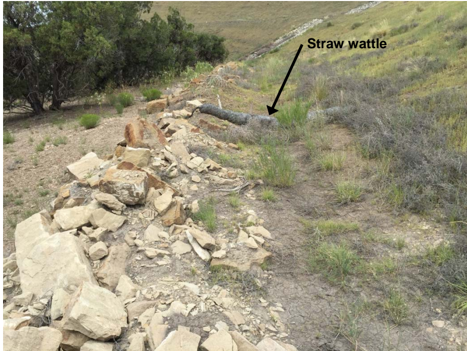
Figure 8: Typical Perimeter Channel Condition
