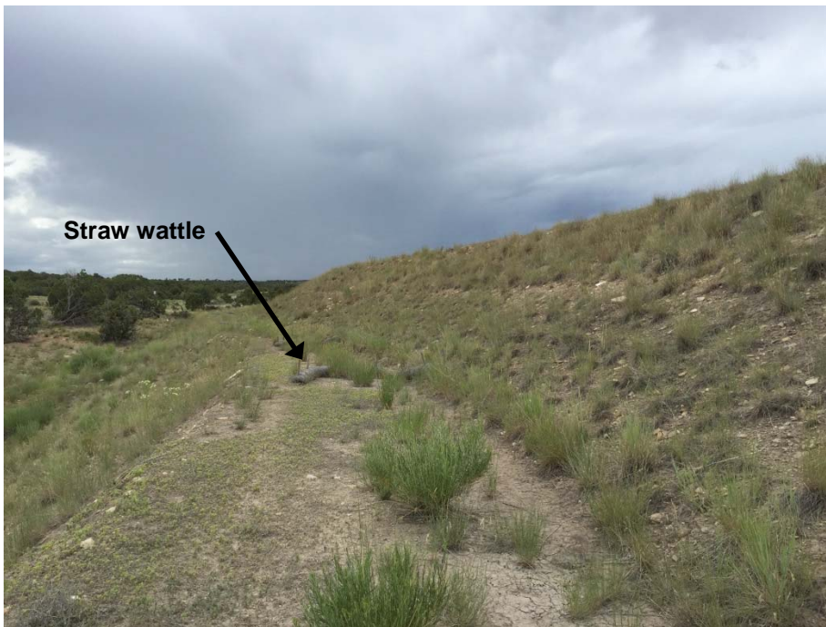
Figure 7: Typical Terrace Channel Condition
