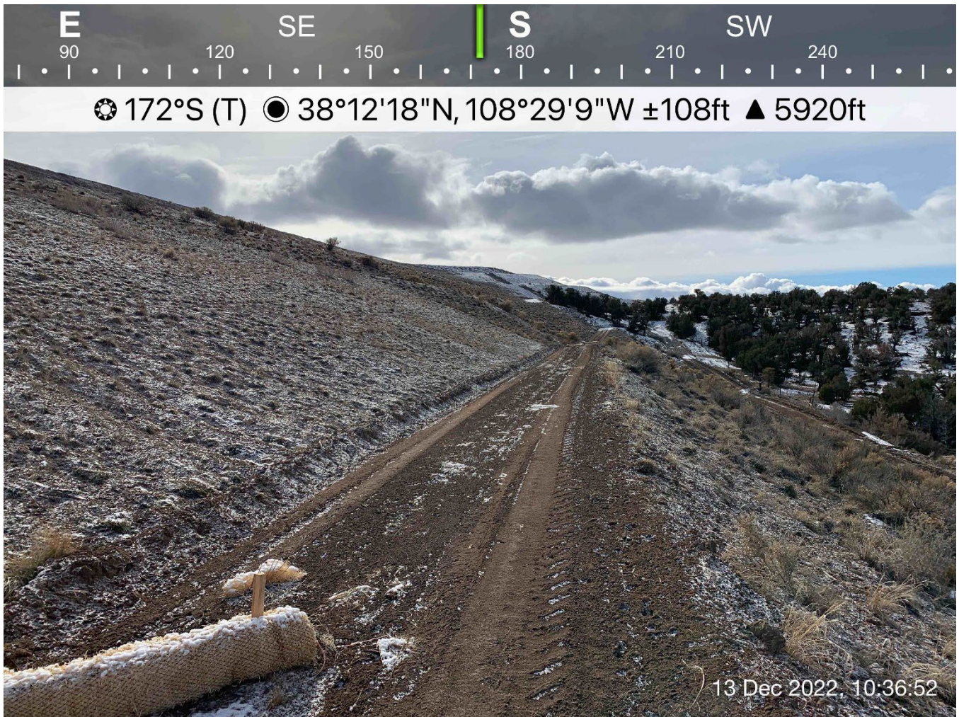
Photograph 8: Typical Condition of Terrace Channels
