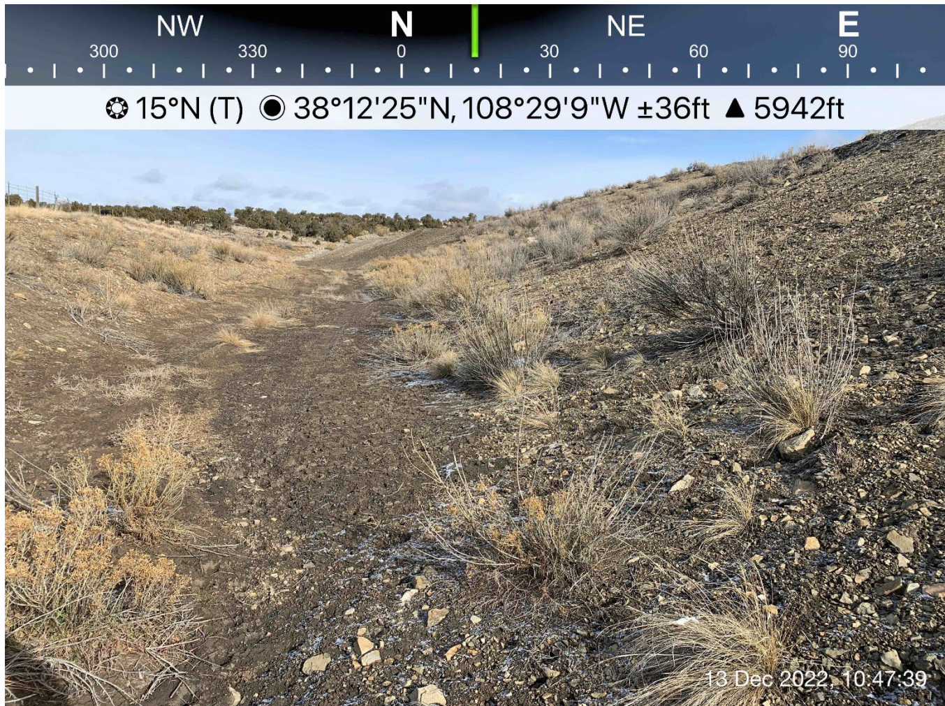
Photograph 6: Typical Condition of Embankment Toes
