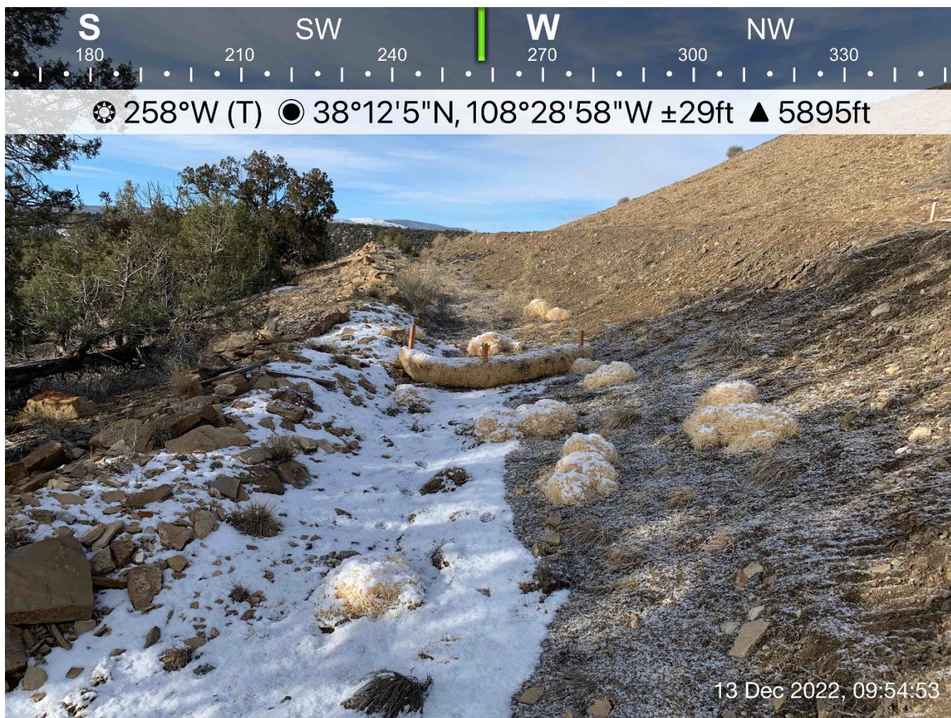
Photograph 9: Typical Condition of Perimeter Channels
