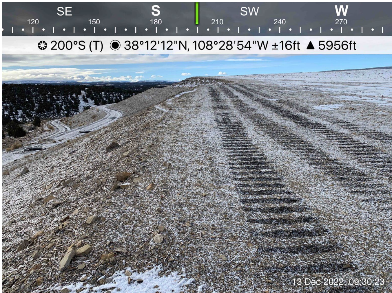
Photograph 2: Typical Condition of Embankment Crests
