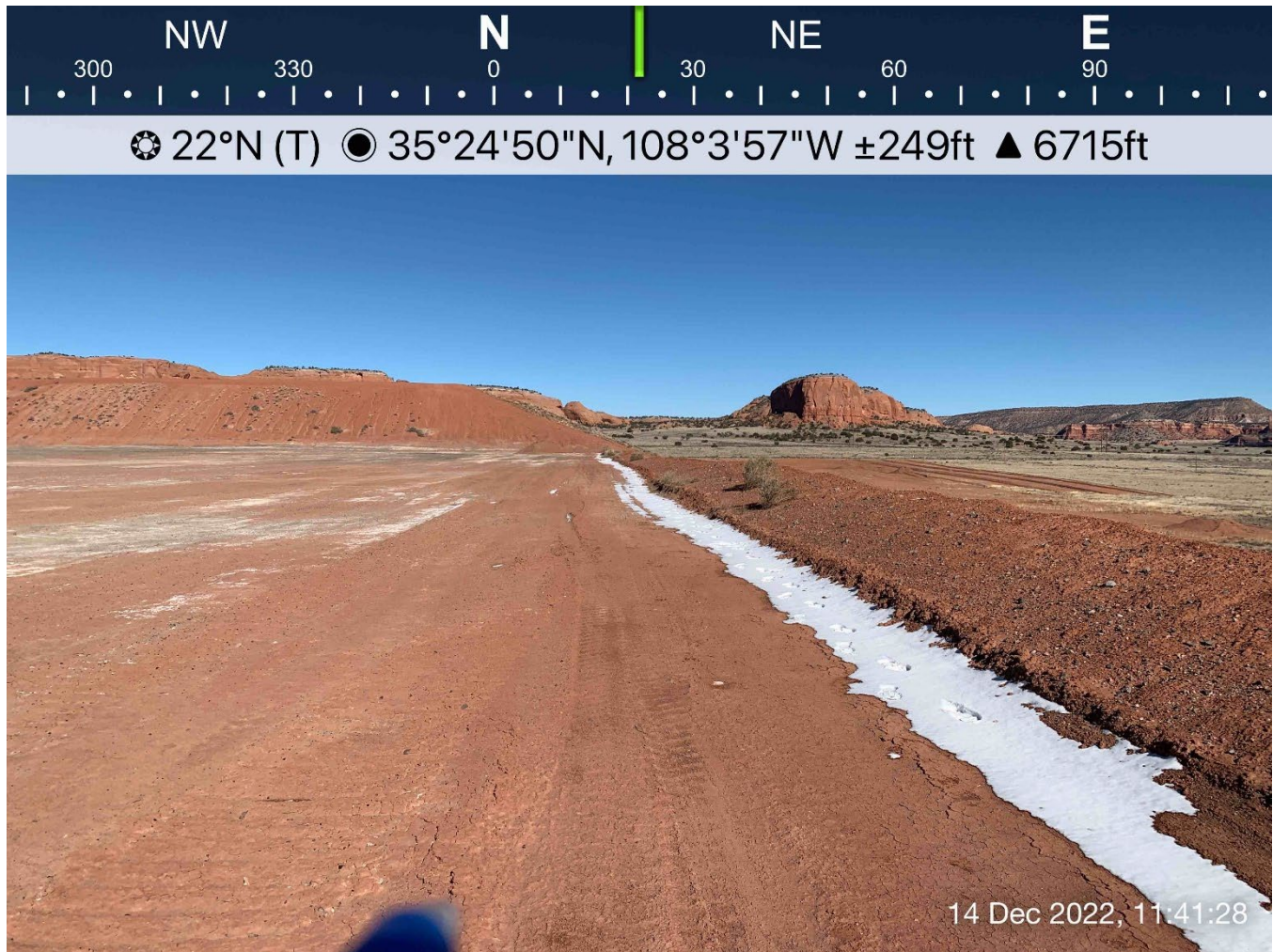
Photograph 2: Typical Condition of Embankment Crest
