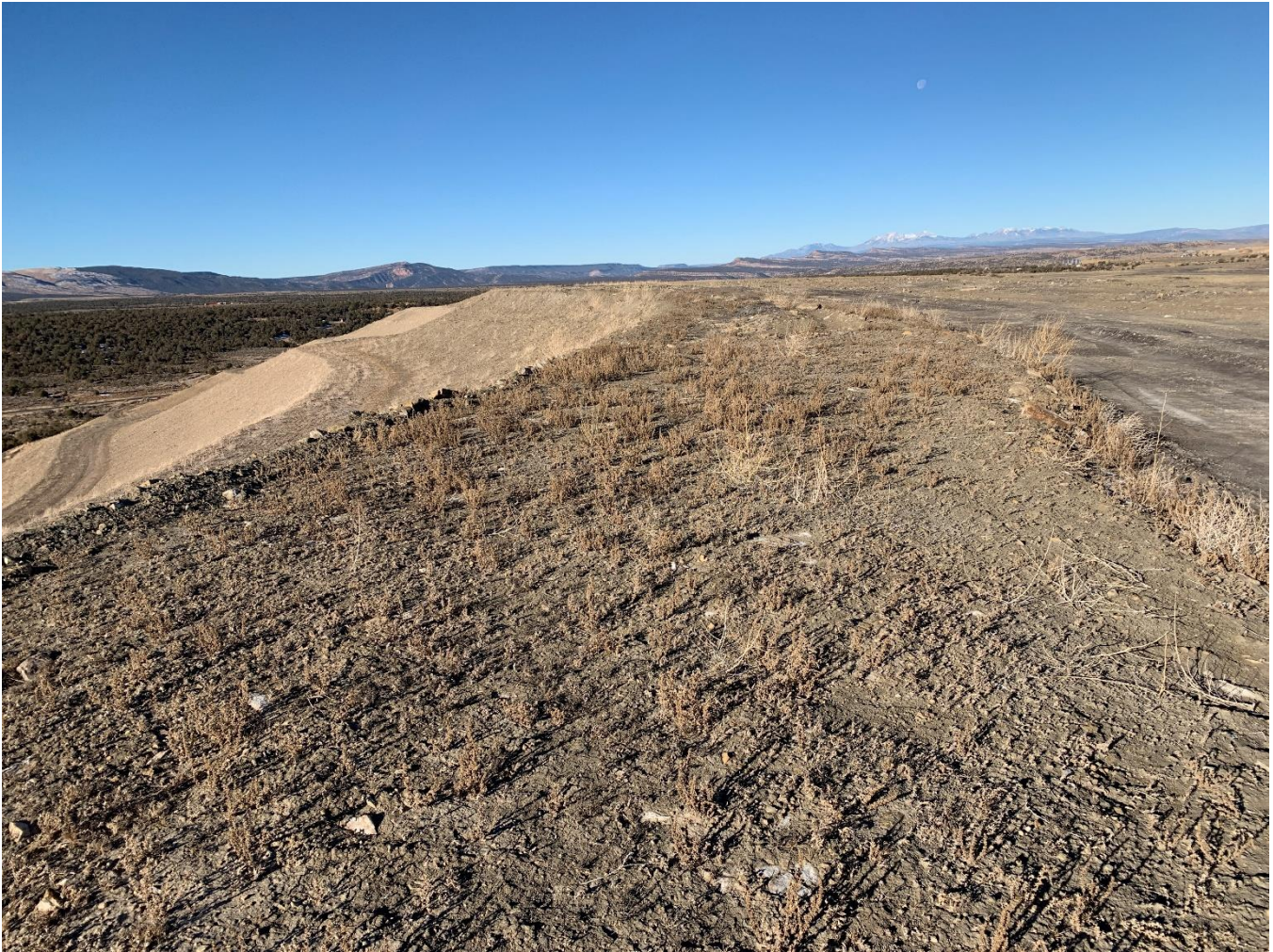
Photograph 2: Typical Embankment Crest Condition
