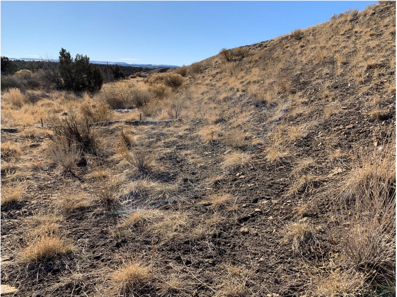
Photograph 4: Typical Embankment Toe Condition
