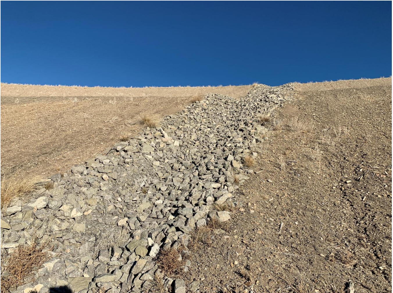
Photograph 5: Typical Downchute Channel Condition
