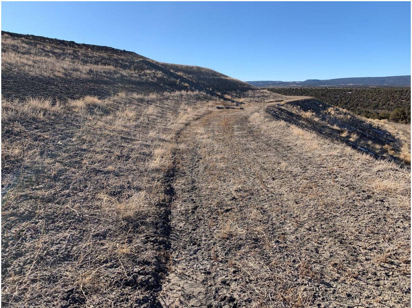
Photograph 6: Typical Terrace Channel Condition
