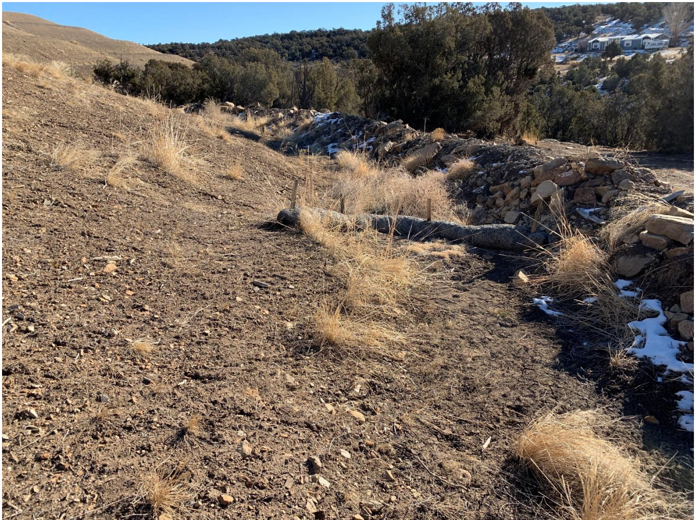
Photograph 7: Typical Perimeter Channel Condition
