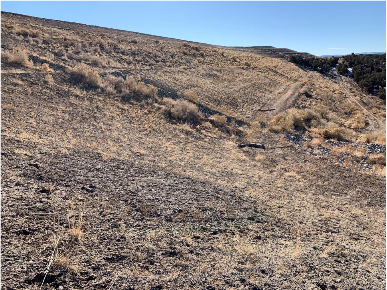
Photograph 3: Typical Embankment Slope Condition
