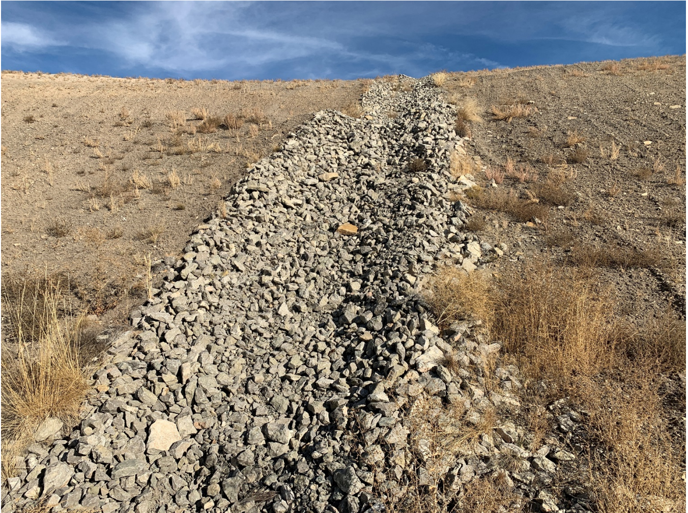
Photograph 5: Typical Downchute Channel Condition
