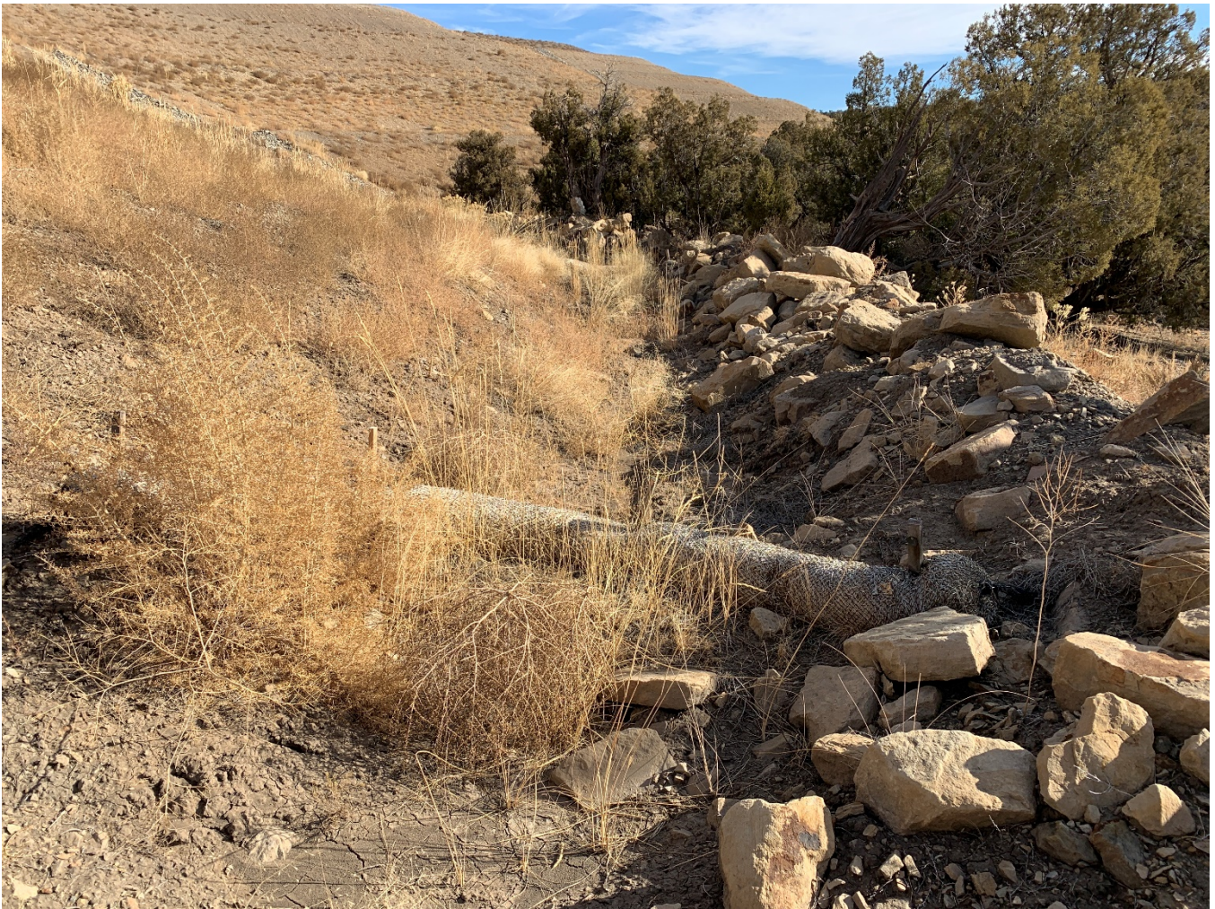
Photograph 7: Typical Perimeter Channel Condition
