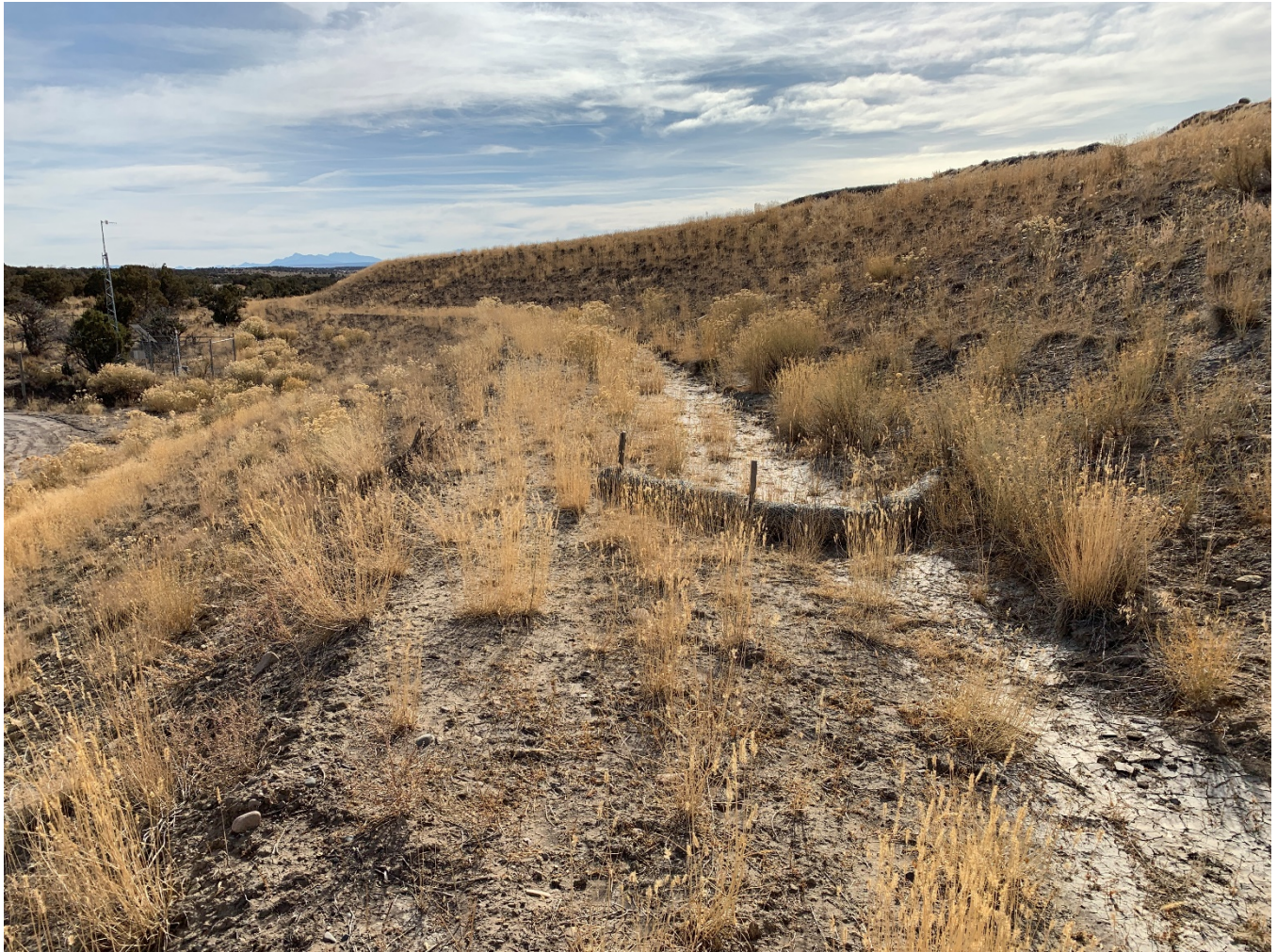
Photograph 6: Typical Terrace Channel Condition
