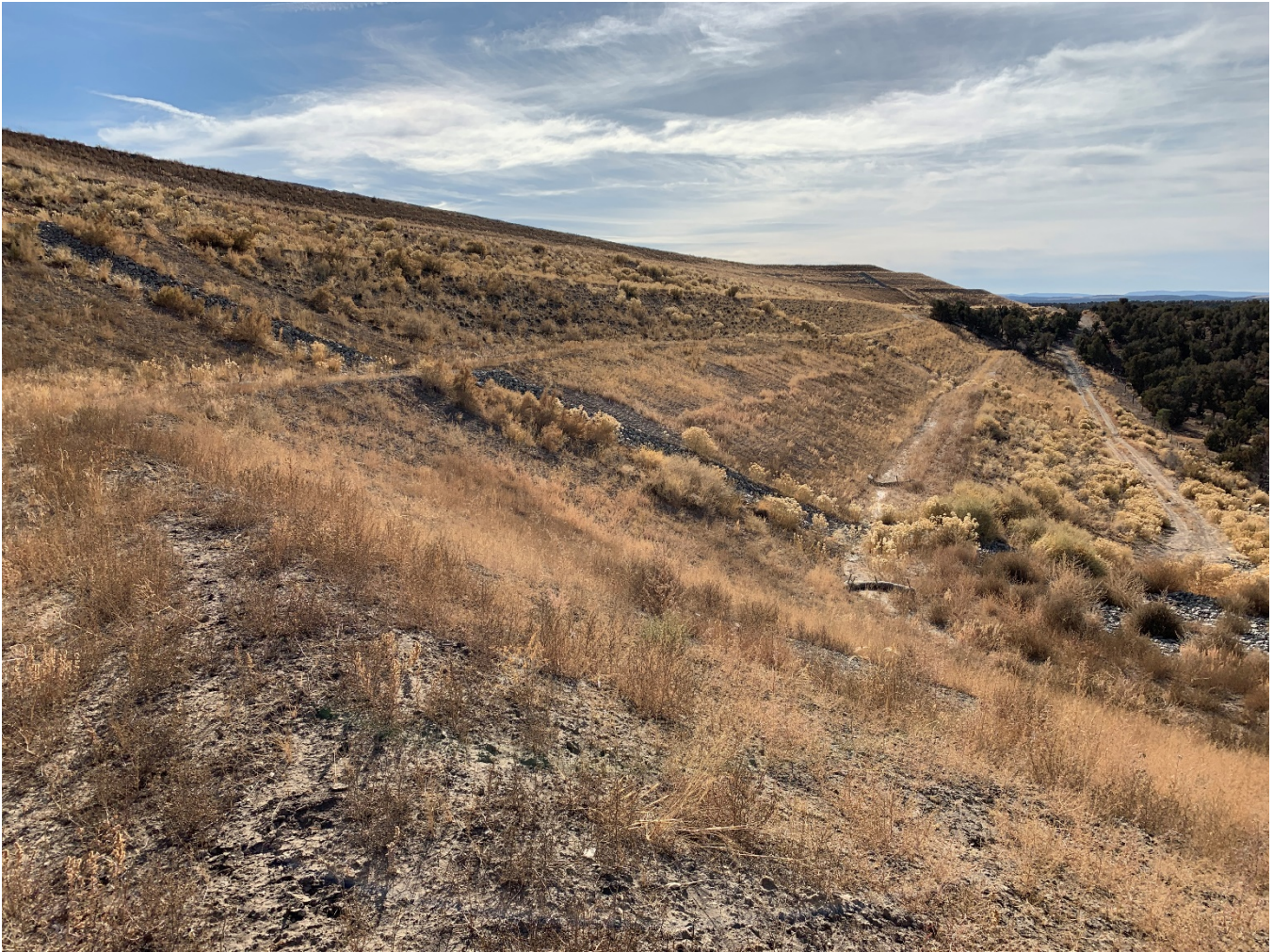
Photograph 3: Typical Embankment Slope Condition
