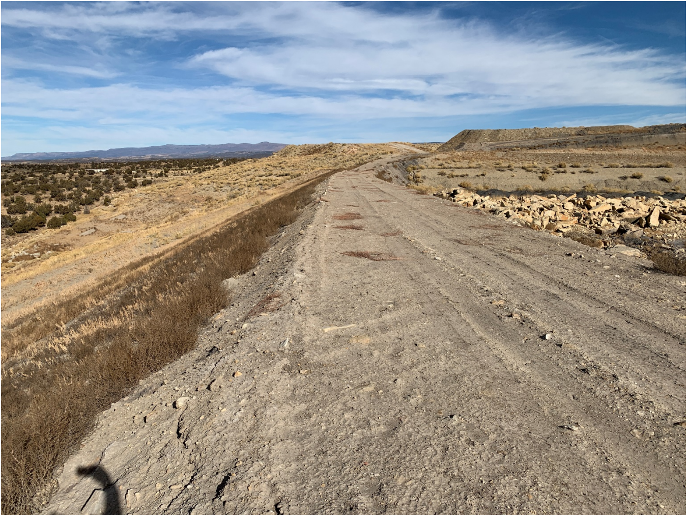
Photograph 2: Typical Embankment Crest Condition
