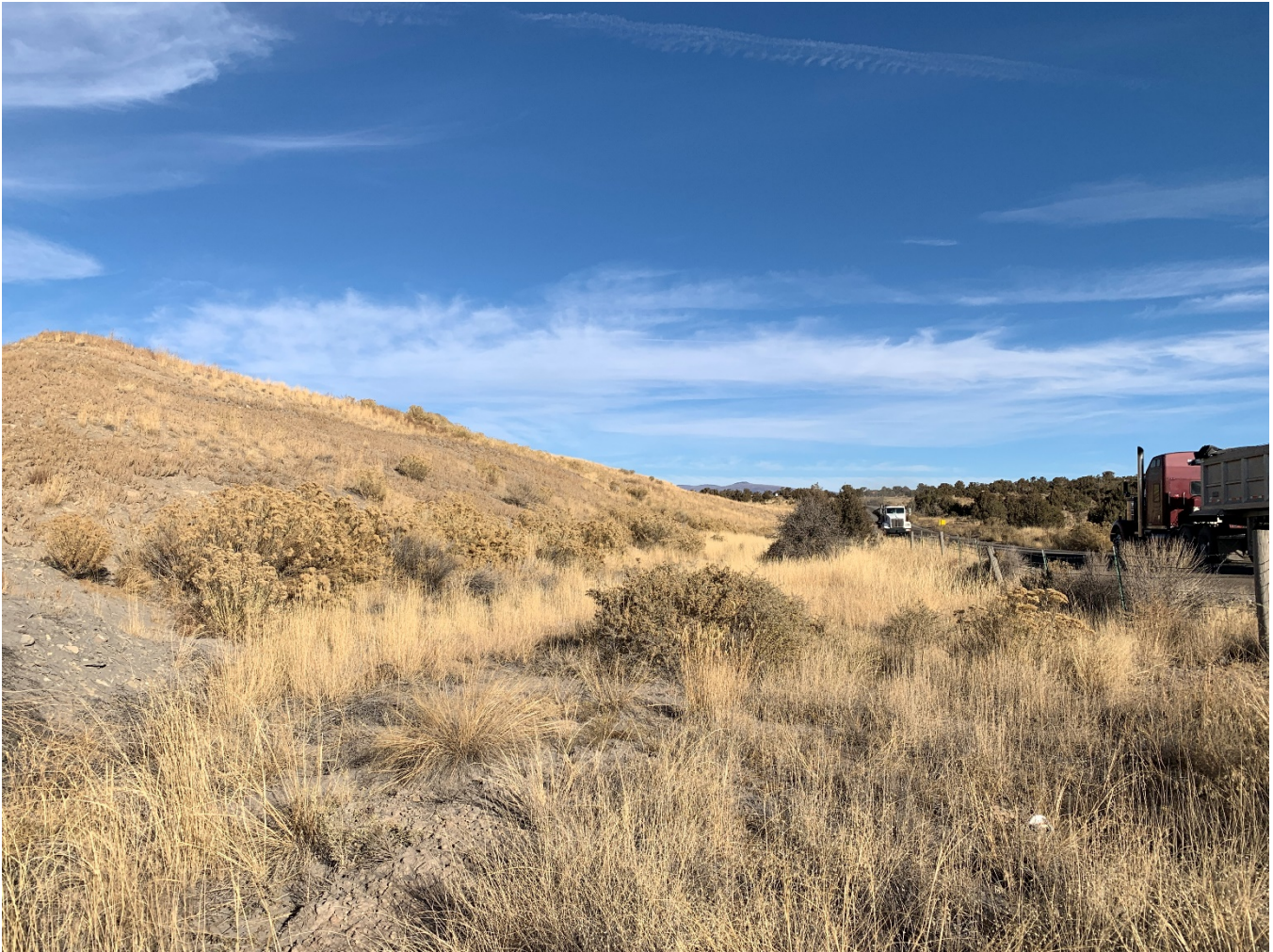
Photograph 4: Typical Embankment Toe Condition
