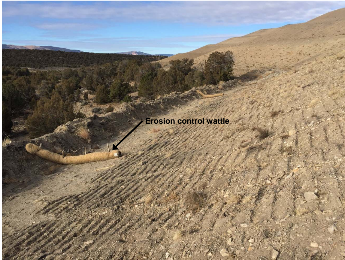
Photograph 7: Typical Perimeter Channel Condition
