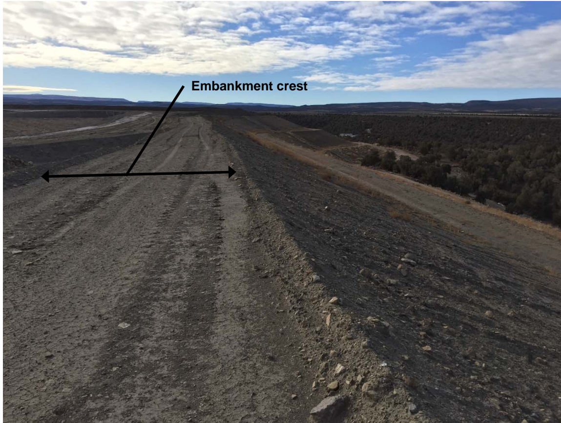
Photograph 2: Typical Embankment Crest Condition
