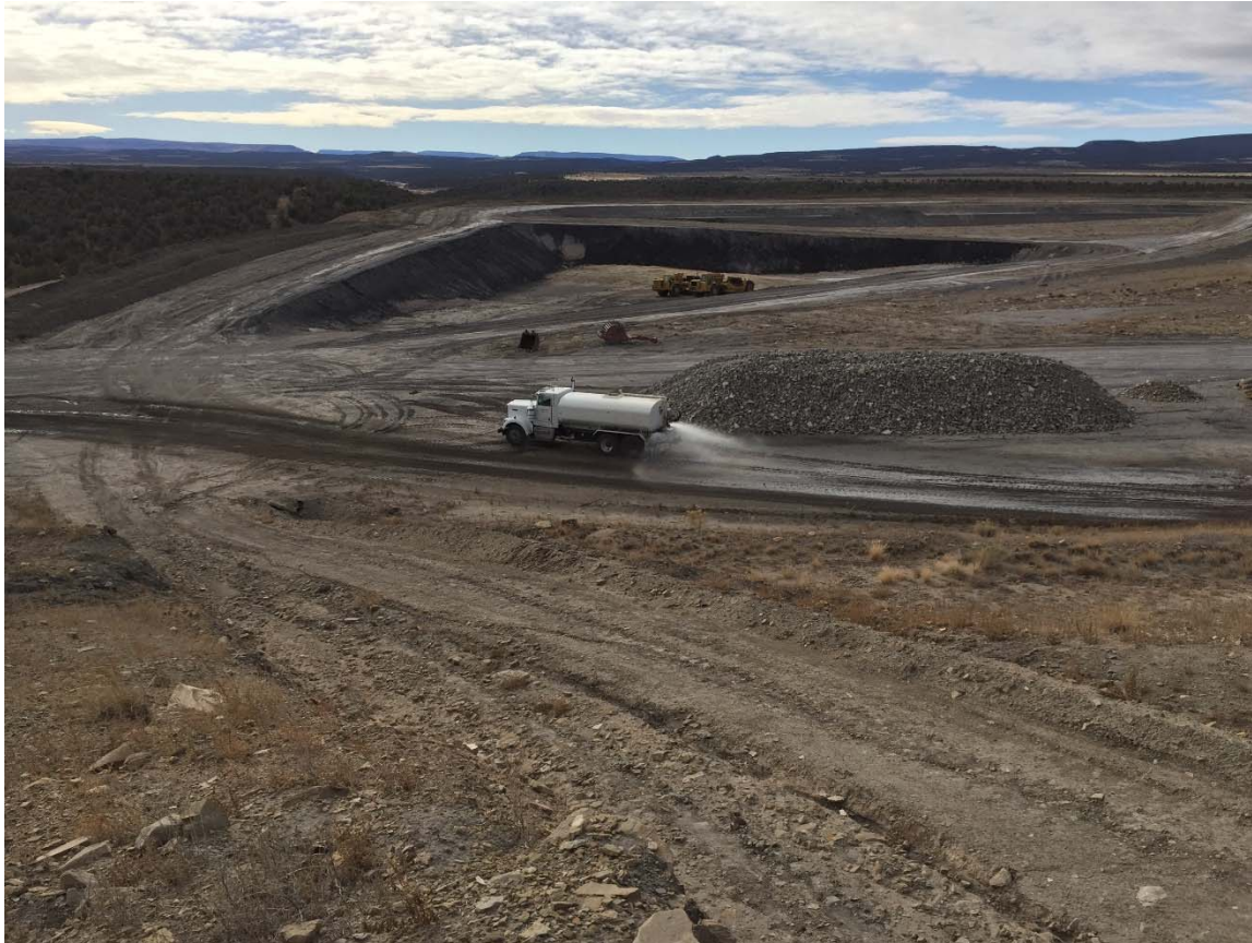
Photograph 1: Typical Ash Deposition Area Condition
