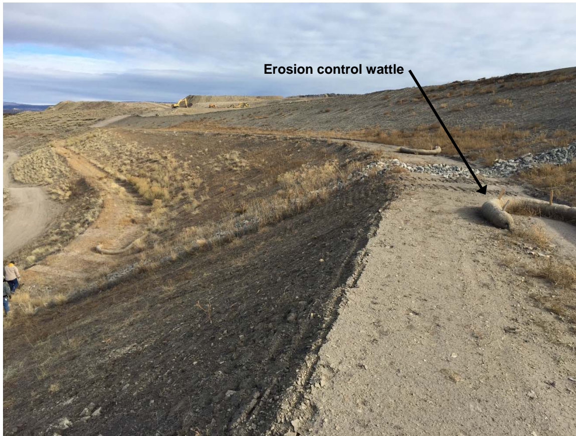
Photograph 6: Typical Terrace Channel Condition
