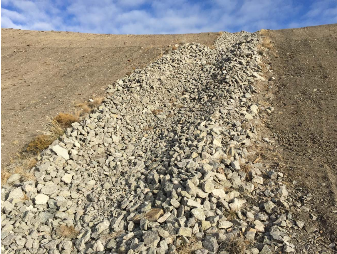
Photograph 5: Typical Downchute Channel Condition
