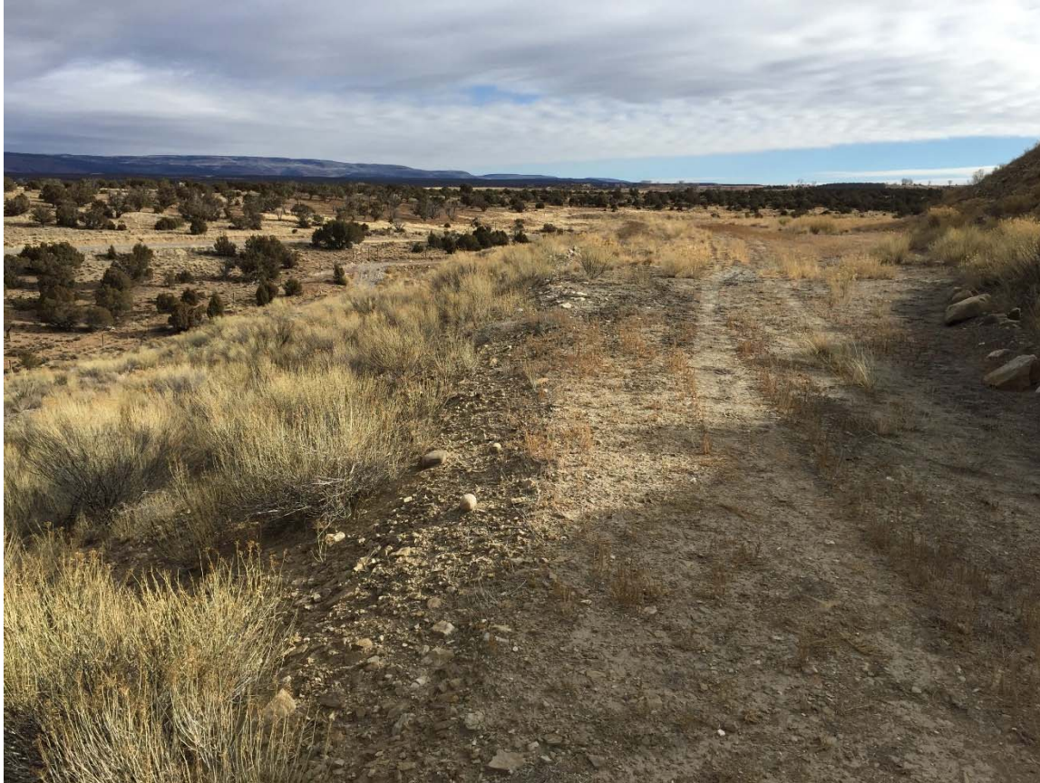
Photograph 4: Typical Embankment Toe Condition
