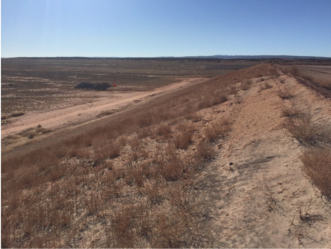
Photograph 4: Typical East Embankment Slope Condition
