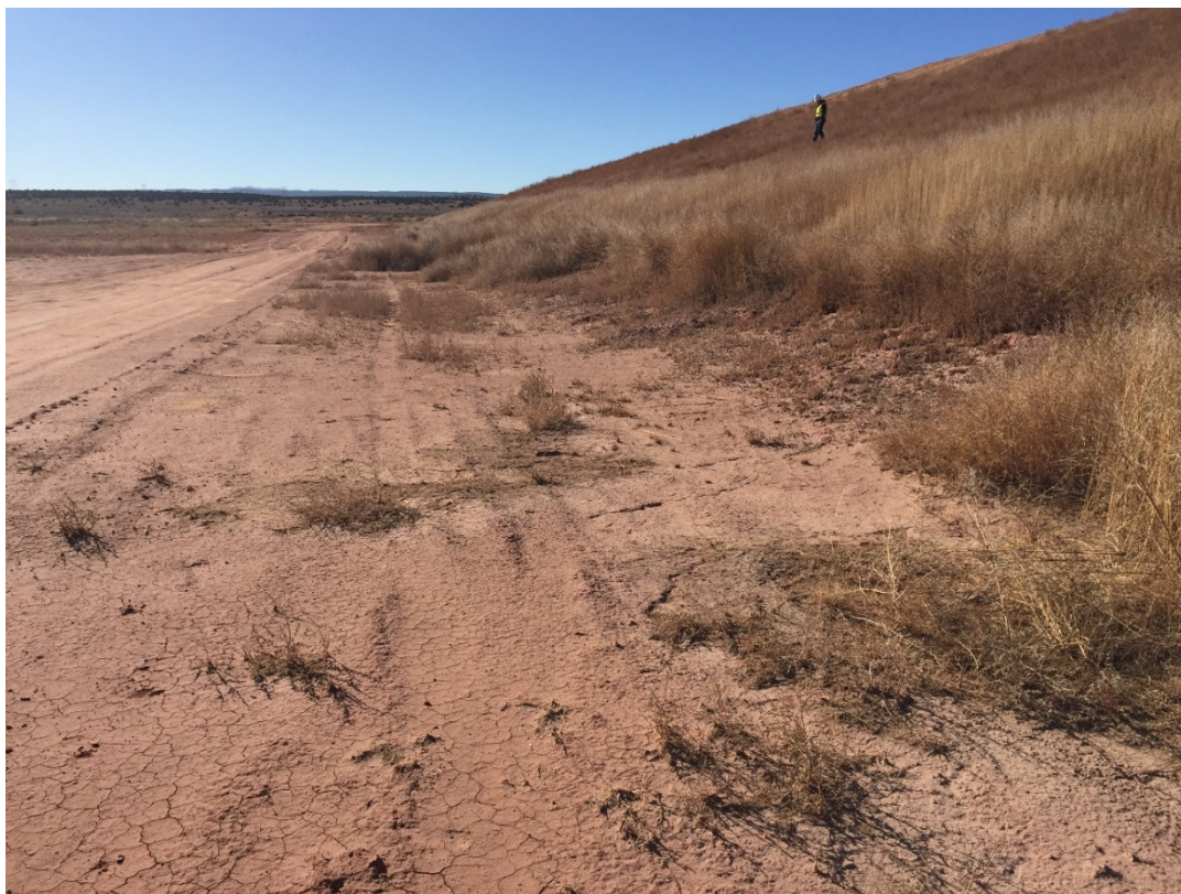
Photograph 7: Typical Embankment Toe Condition
