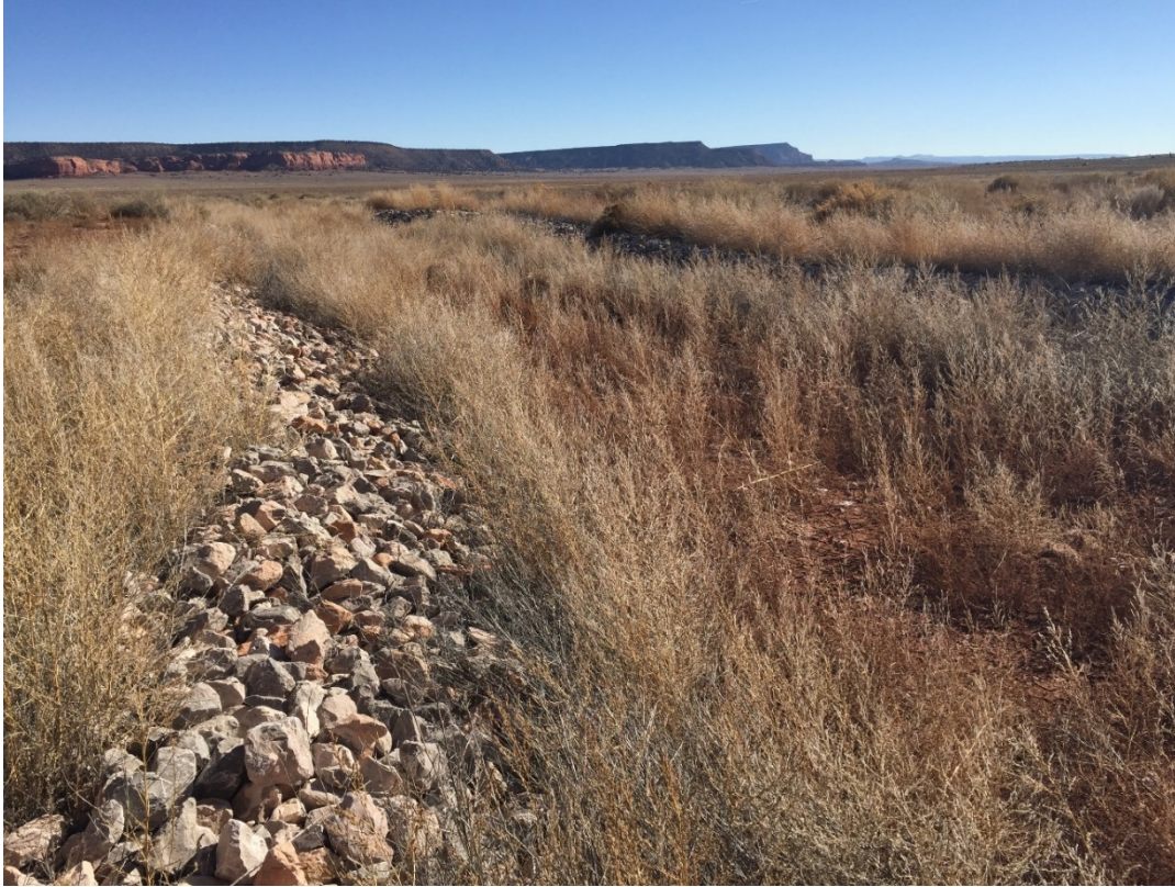
Photograph 8: Typical Storm Water Channel Condition
