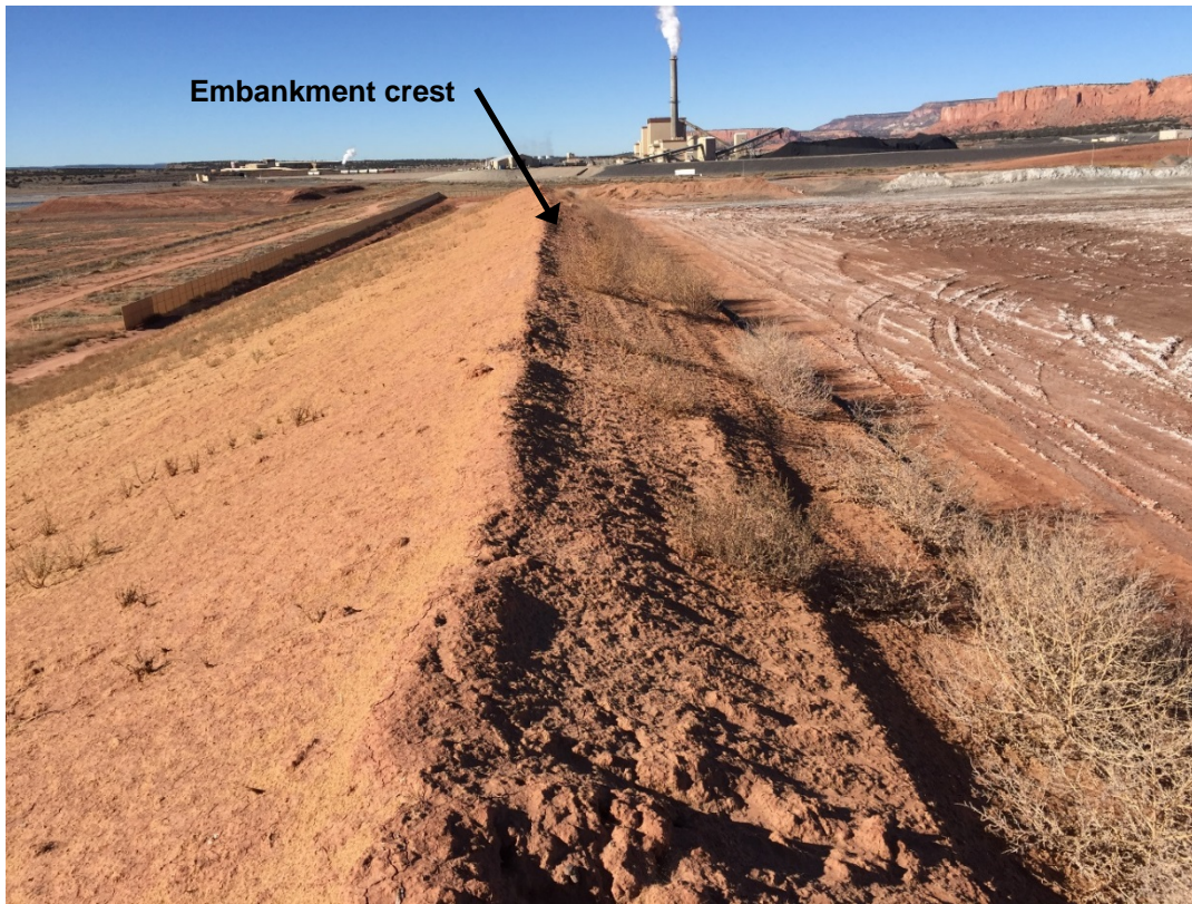
Photograph 3: Typical Embankment Crest Condition
