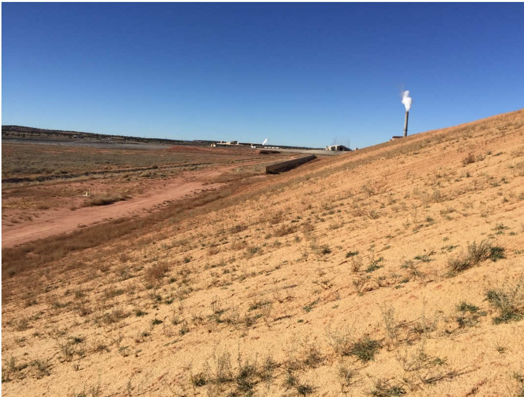
Photograph 6: Typical South Embankment Slope Condition
