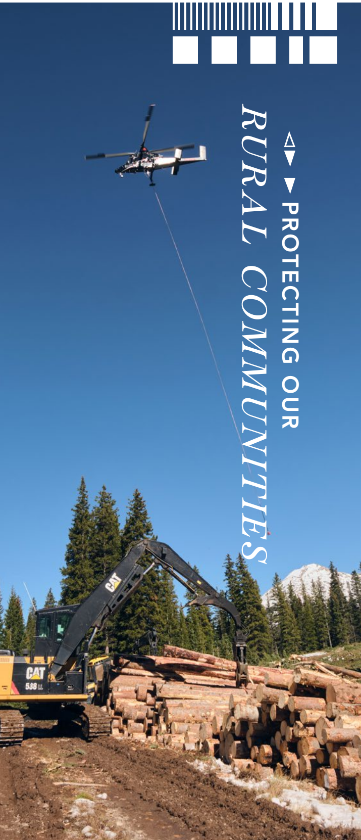
Heli-logging in Silverton, CO to help reduce wildfire risks.
