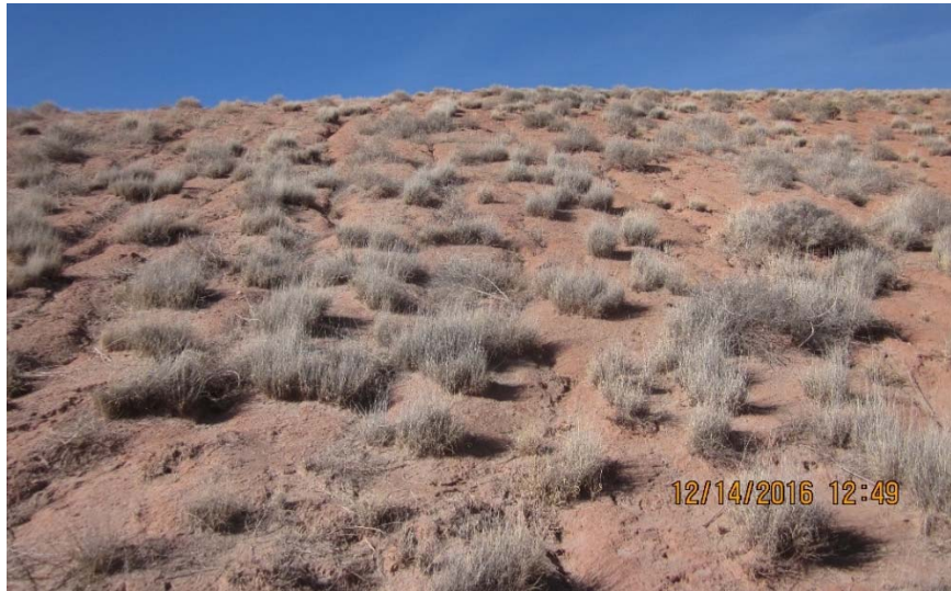
Figure 4: Typical East-embankment Slope Condition
