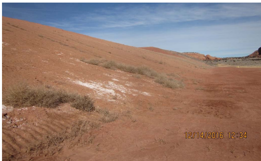
Figure 6: Typical Embankment Toe Condition
