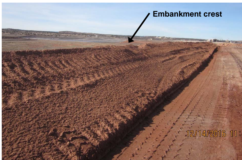
Figure 3: Typical Embankment Crest Condition
