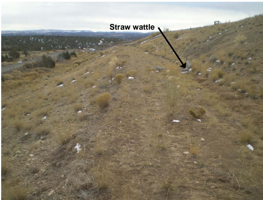
Photograph 7: Typical Terrace Channel Condition
