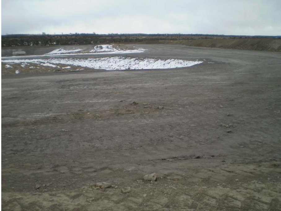
Photograph 1: Typical Ash Deposition Area Condition
