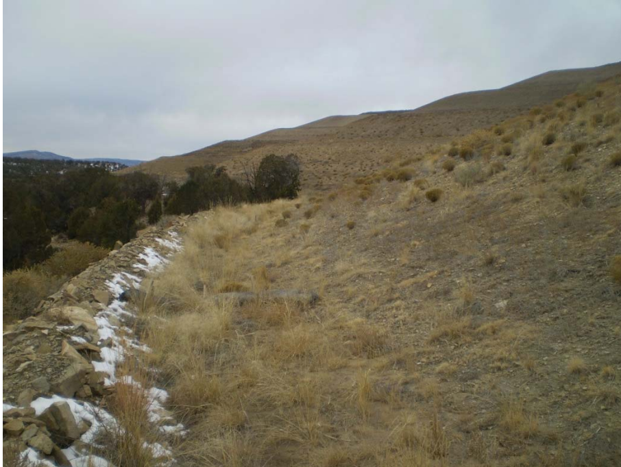
Photograph 5: Typical Embankment Toe Condition
