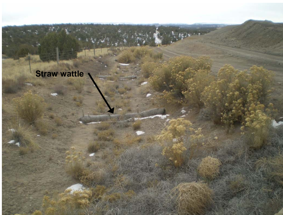
Photograph 8: Typical Perimeter Channel Condition
