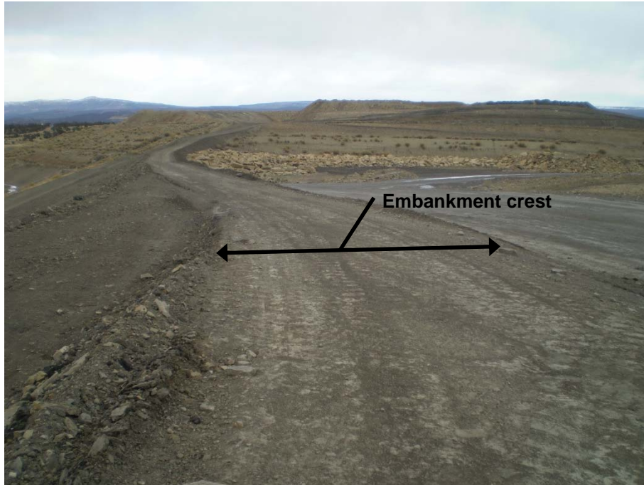
Photograph 2: Typical Embankment Crest Condition
