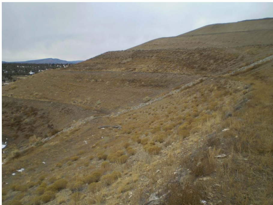
Photograph 3: Typical Embankment Slope Condition
