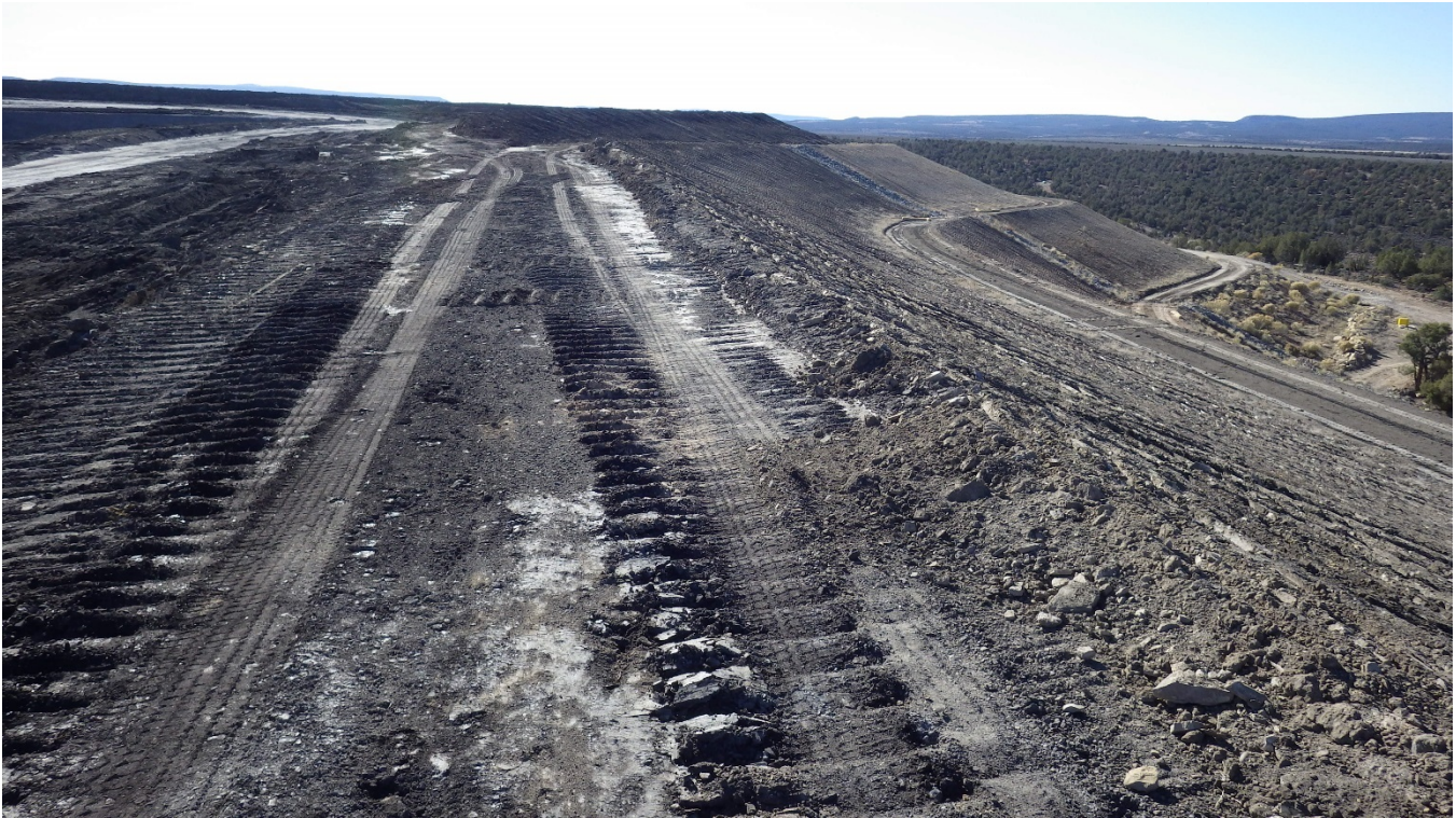
Photograph 2: Typical Embankment Crest Condition
