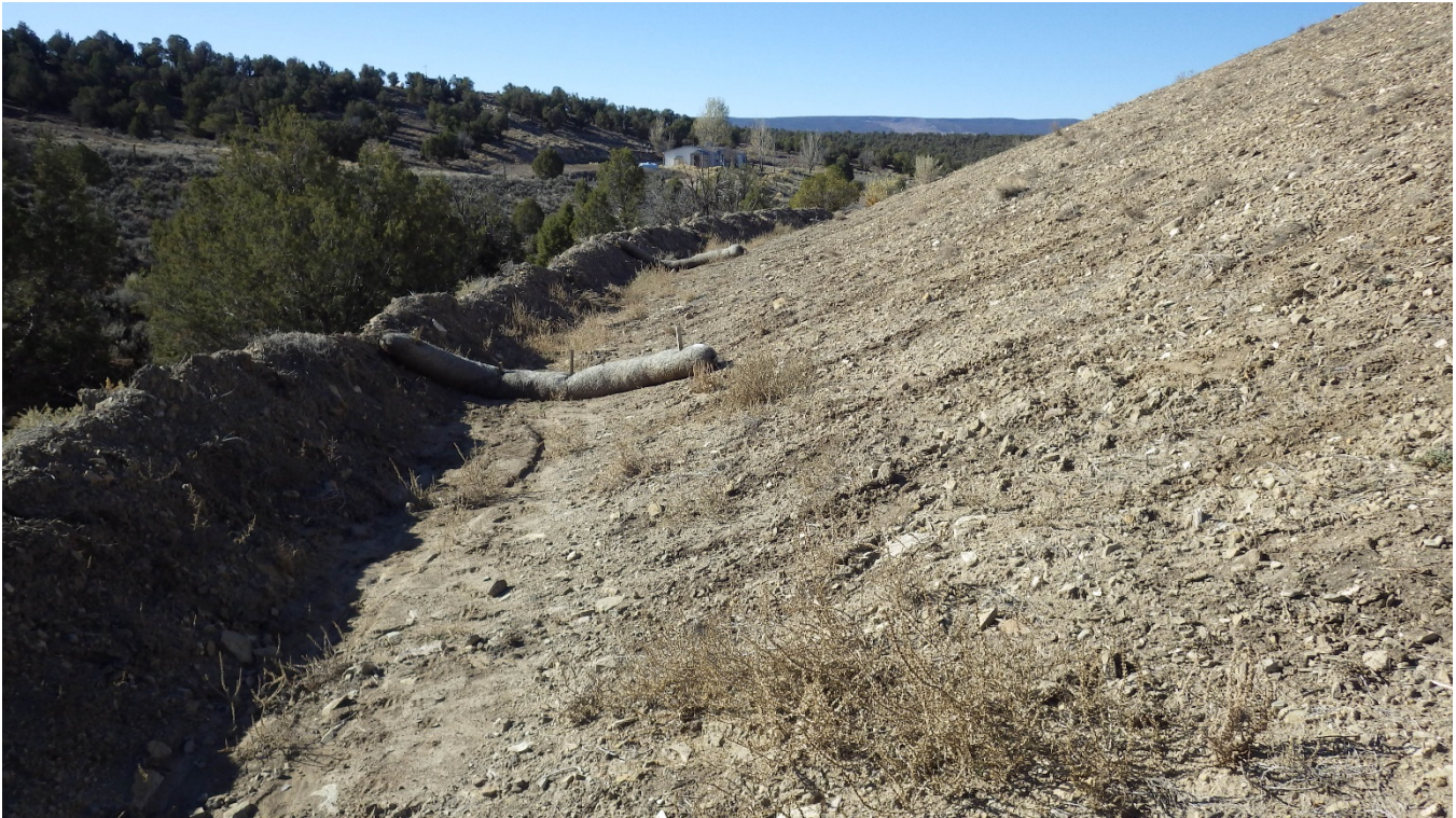
Photograph 7: Typical Perimeter Channel Condition
