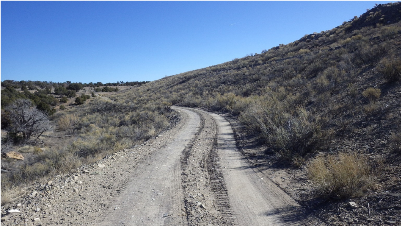
Photograph 4: Typical Embankment Toe Condition
