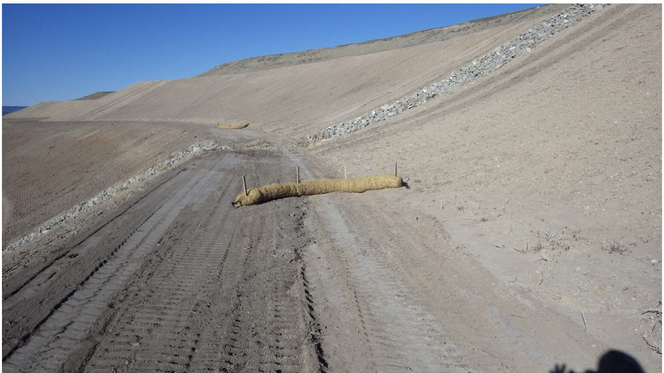
Photograph 6: Typical Terrace Channel Condition
