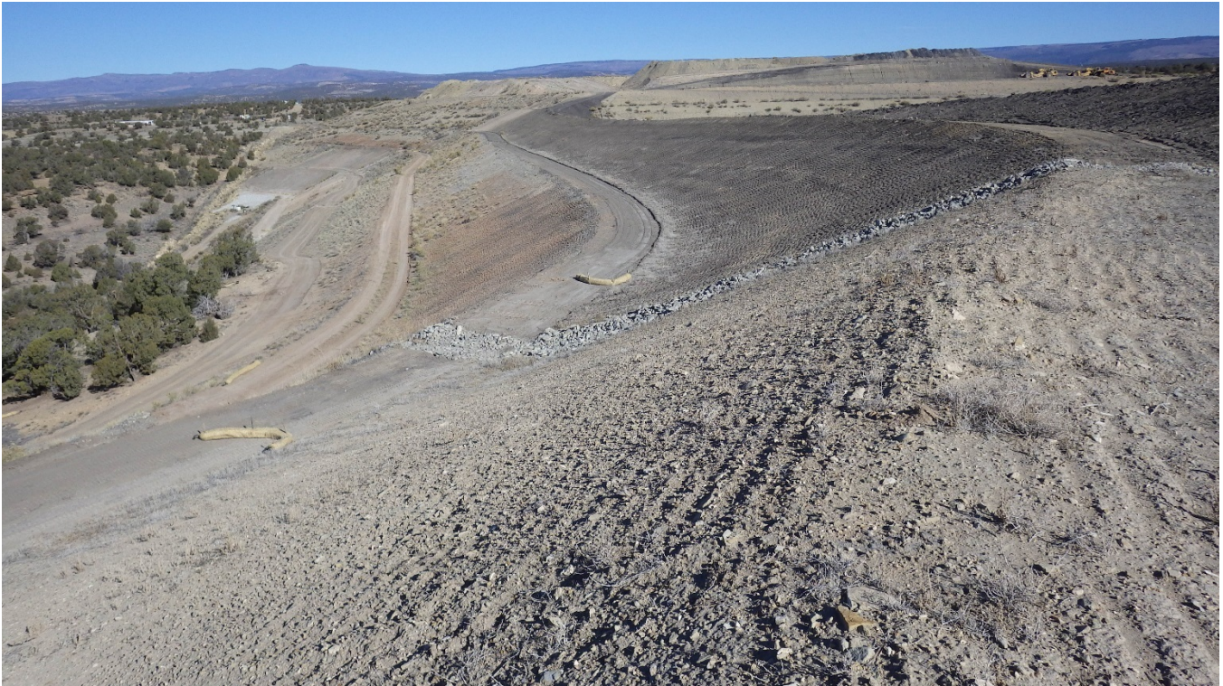
Photograph 3: Typical Embankment Slope Condition
