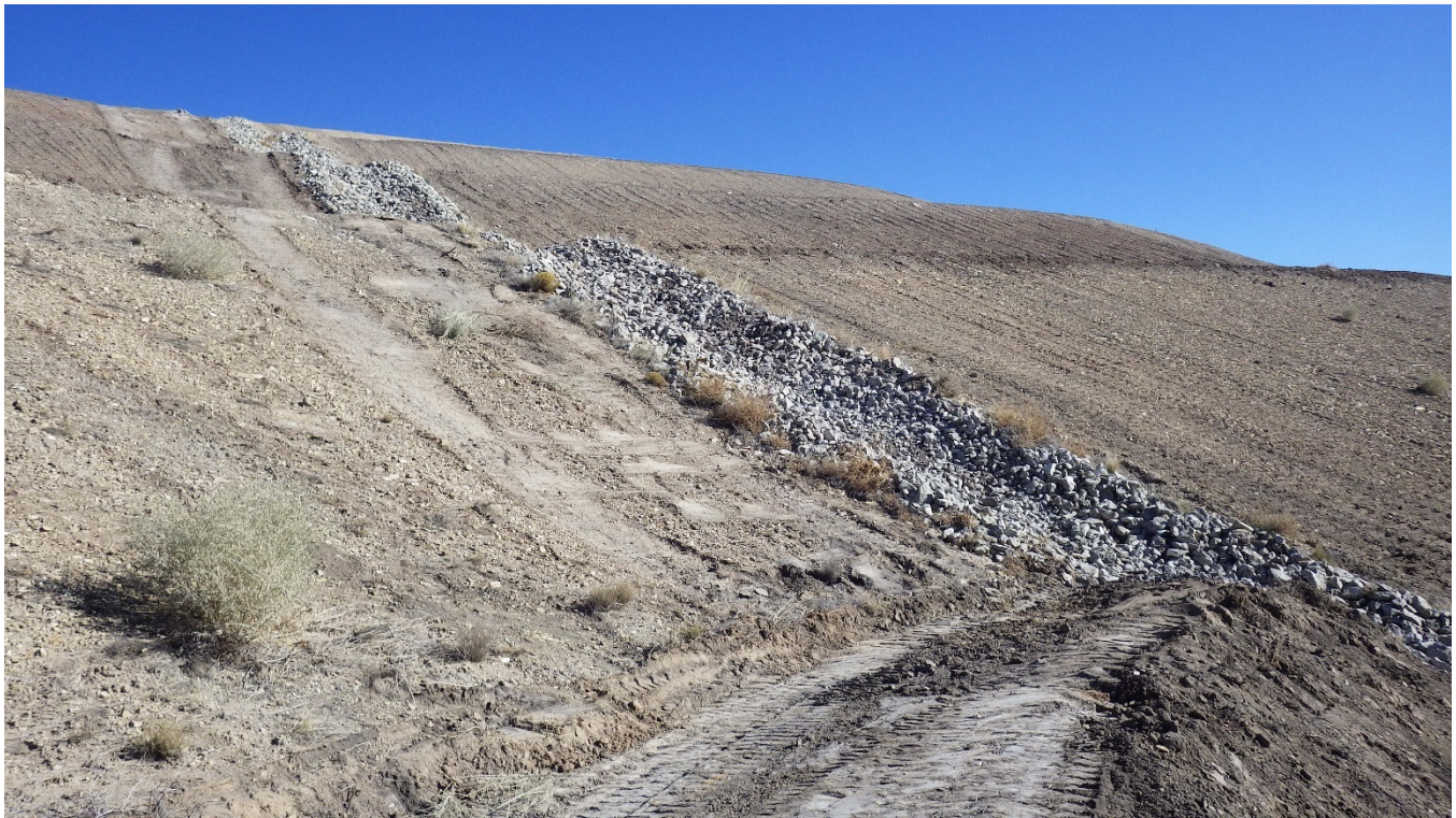
Photograph 5: Typical Downchute Channel Condition
