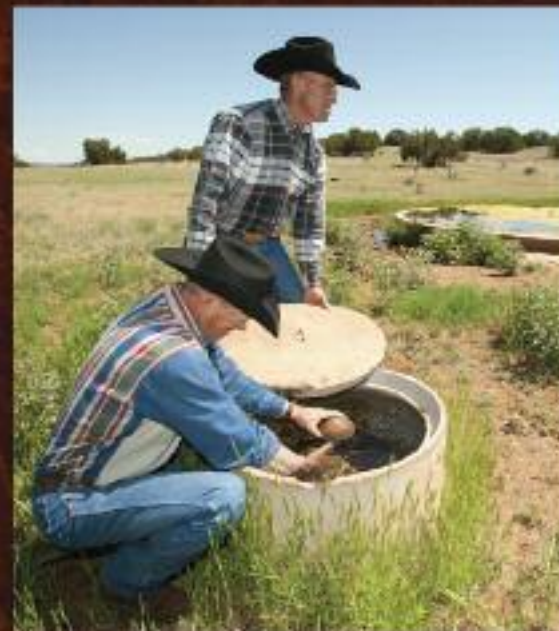
Nephew Steve Woonten (top) assists John in checking float valves on one of the many water tanks on the ranch.
